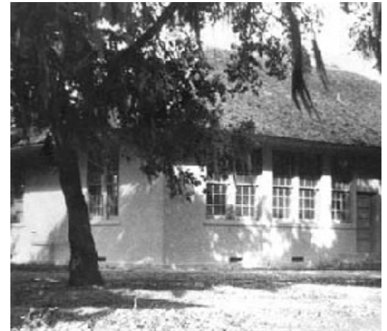
DO YOU REMEMBER THIS BUILDING? It is one of Spring Branch School District's first school houses. It now stands on the campus of Spring Branch Elementary School and is used for the entire school system because of its historical significance. About 50 pupils attend the school.
