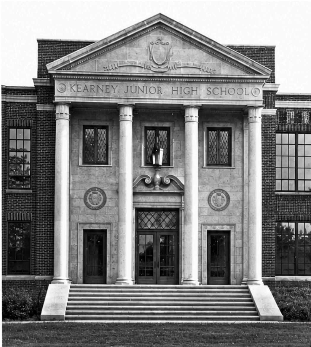
MAIN ENTRANCE DETAIL.
