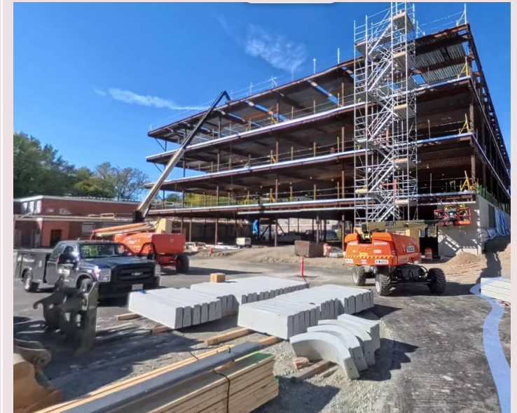
Structural steel (south elevation)
