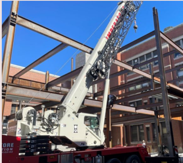
Steel erection at addition ongoing
