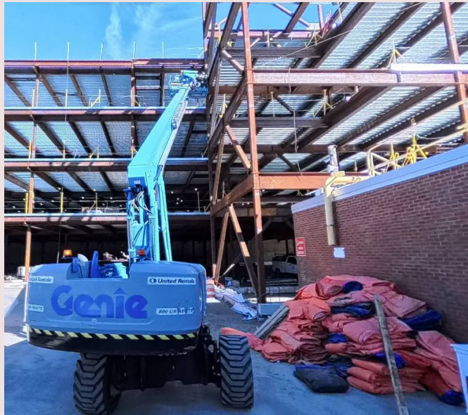
Structural steel (west elevation)
