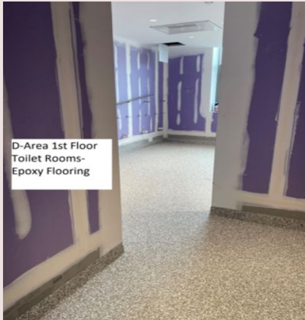
D-Area 1st FL Toilet Rooms - Epoxy Flooring
