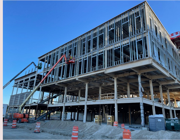
Exterior wall framing
