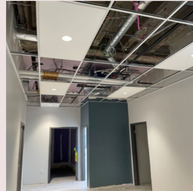
D-Area 1st FL ceiling grid install and painting started
