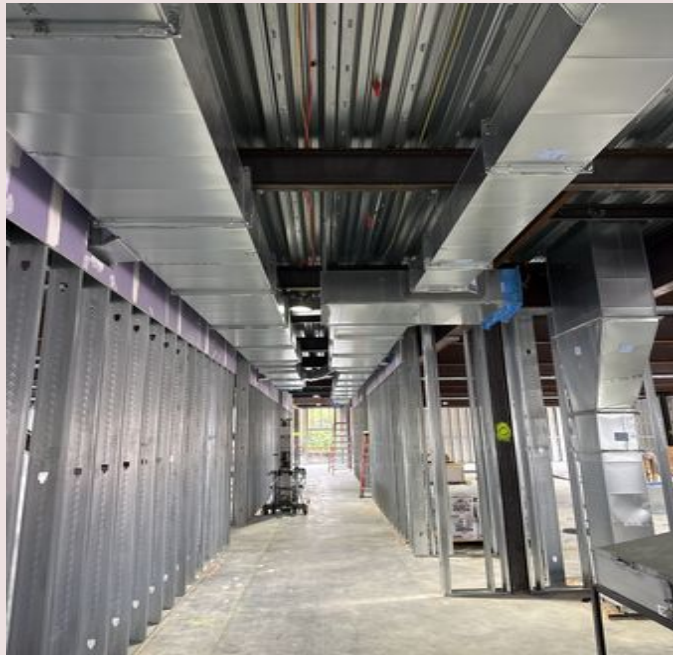
Interior wall and ductwork installation
