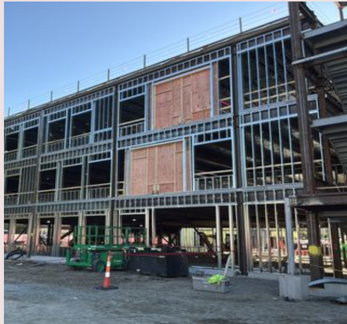
Exterior wall framing
