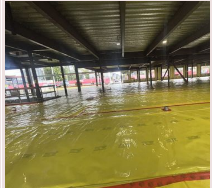
Area 1: Slab on grade preparation
