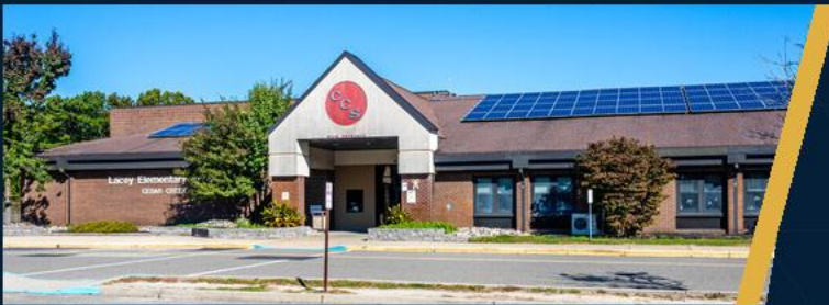
CCS Cedar Creek Elementary School
