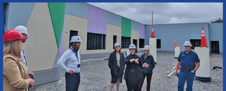
Members of the Special Education Advisory Council tour the Expansion site and learn more about the specialized learning spaces and interior courtyards.
