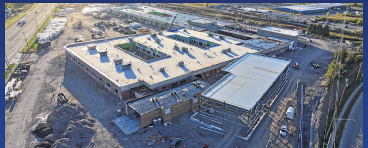
Construction on the Erie 1 BOCES Instructional Services Expansion project continues to progress steadily, with foundations and siding now in place for all six courtyards and the gymnasium spaces, further bringing the vision for the new campus to life.
