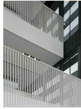
slat railing - typical
