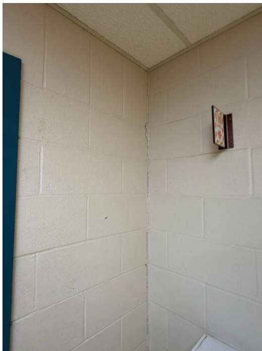
Interior CMU block separation and cracks
