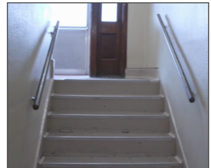
The building has several elevation changes and only a lift located on one side of the building that does not go to the third floor.
