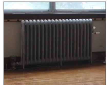
Classroom radiators have leaked and damaged the supporting beams on the 3rd floor, deeming spaces unusable.
