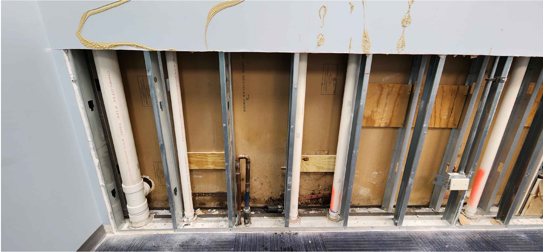
EXISTING PIPING IN PLUMBING WALL - BATHROOM 115A
