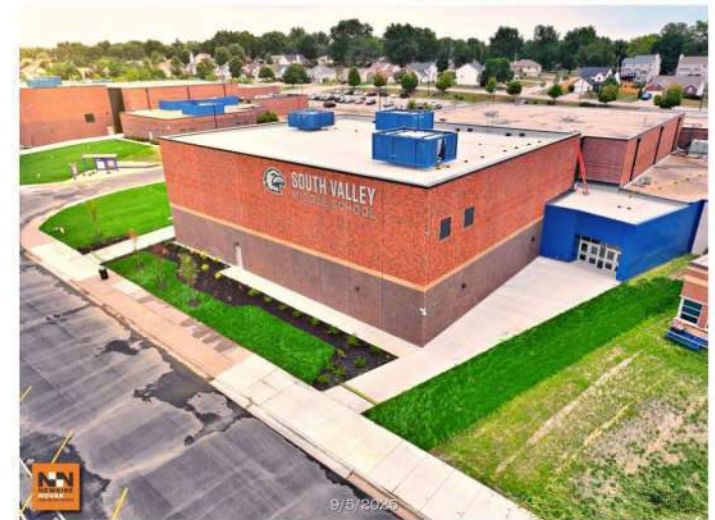
SVMS Exterior View
