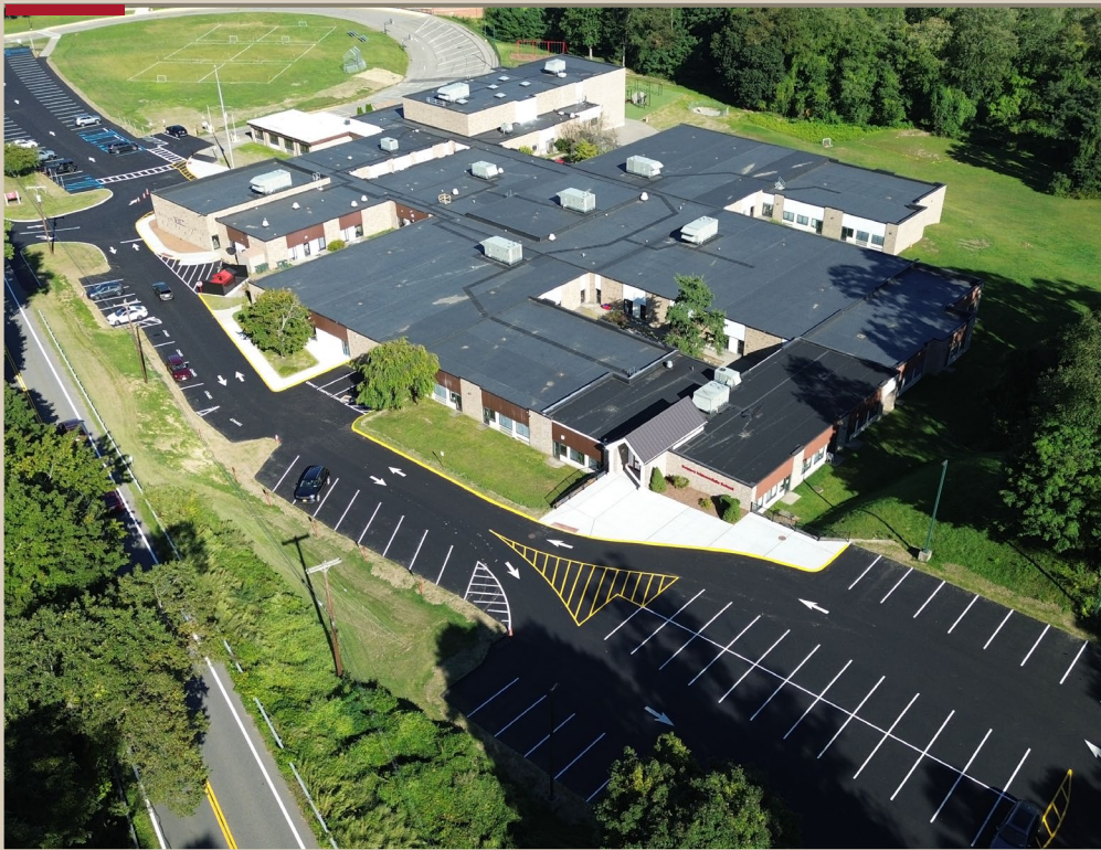
AERIAL VIEW OF NEW SIS SITEWORK
