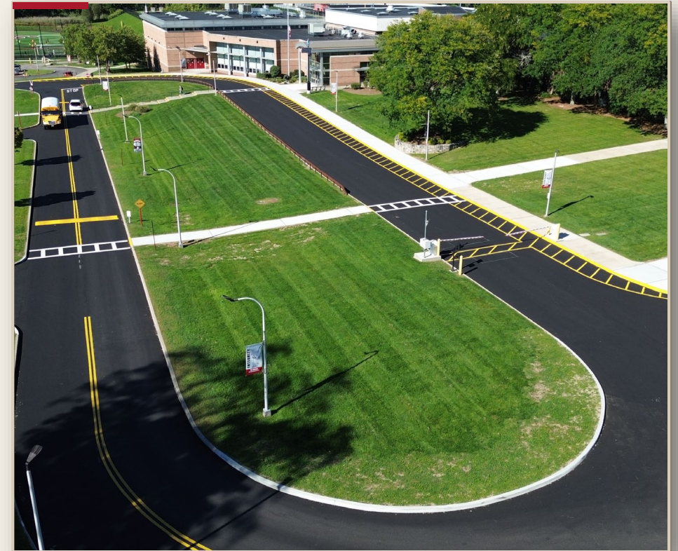
AERIAL VIEW OF NEW SHS SITEWORK PHOTO
