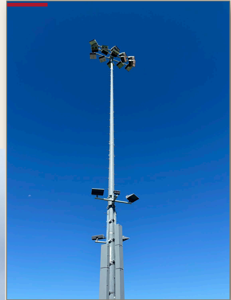
NEW LIGHT FIXTURES INSTALLED ON TURF #1 AT SHS
