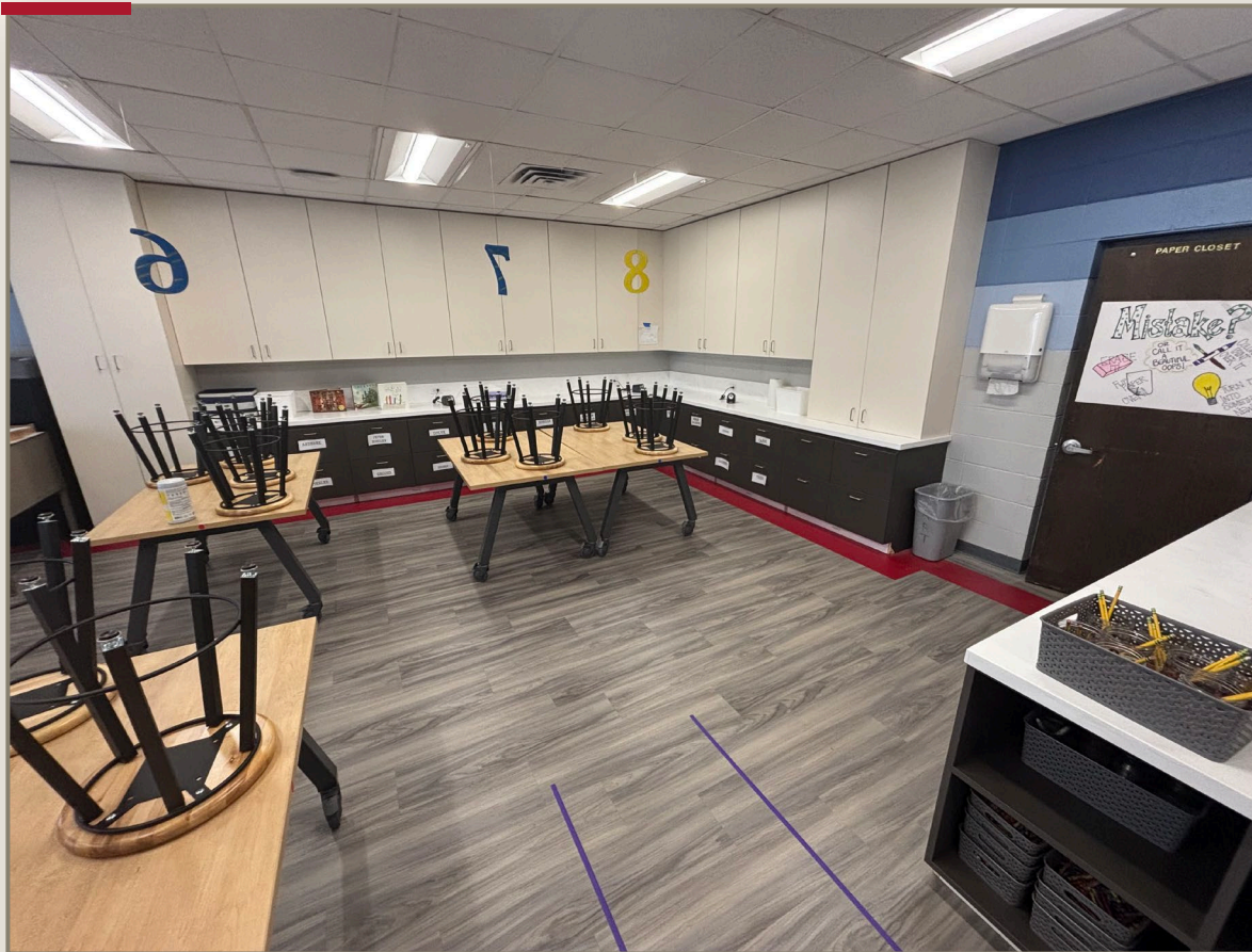
NEW CASEWORK AND FLOORING INSTALLED IN SIS ART ROOM
