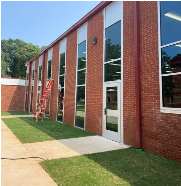
Installation of new storefront windows at cafeteria
