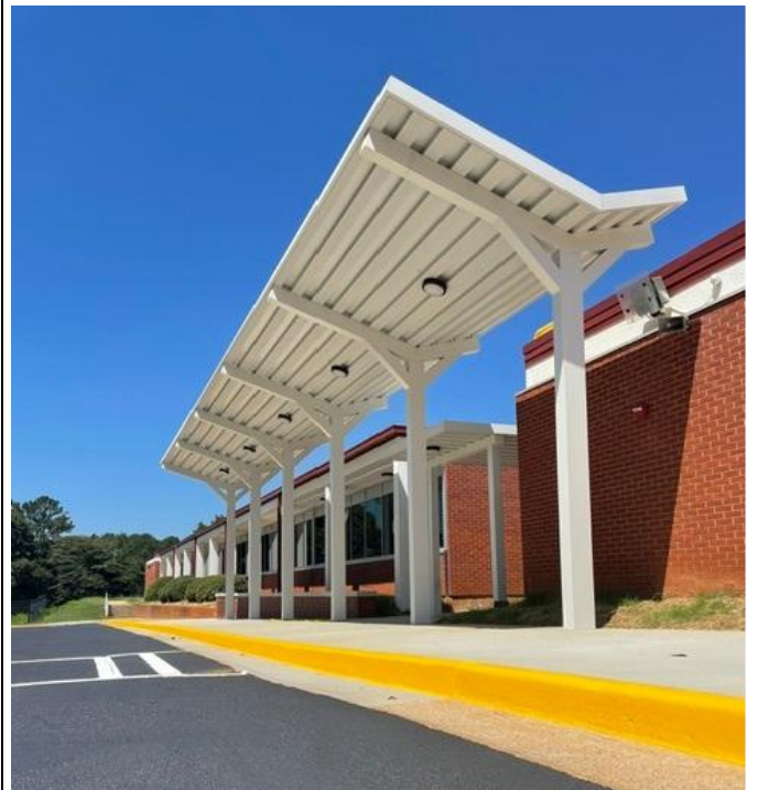
Installation of new bus canopy
