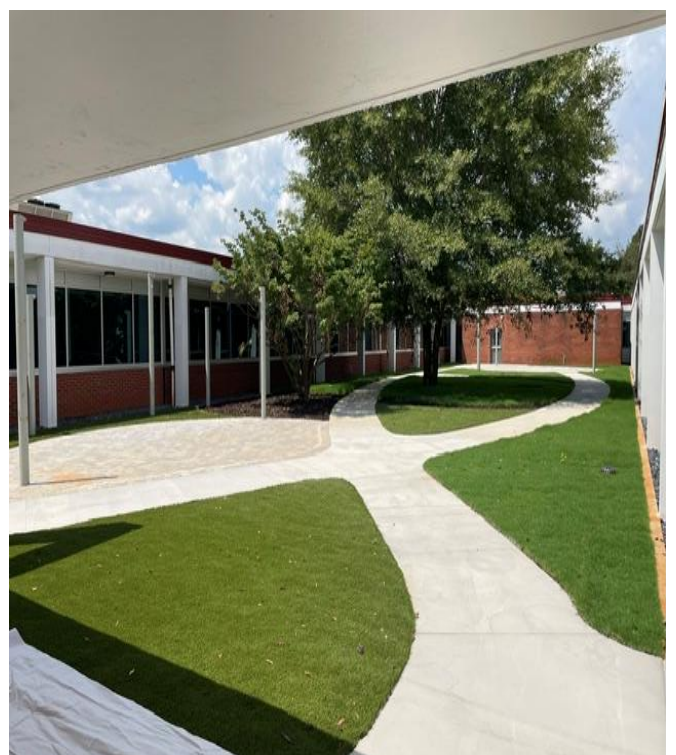
Installation of hardscapes at courtyard
