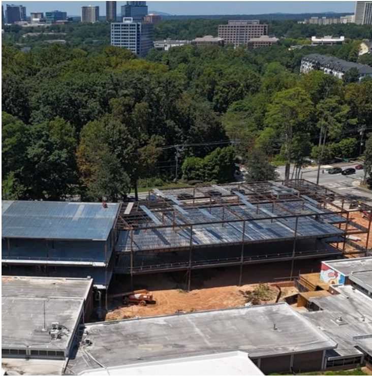
Steel erection at 3 story addition
