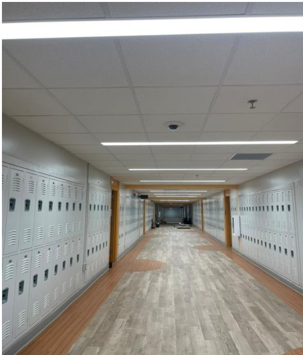
New flooring, paint, ceiling grid at 100 corridor
