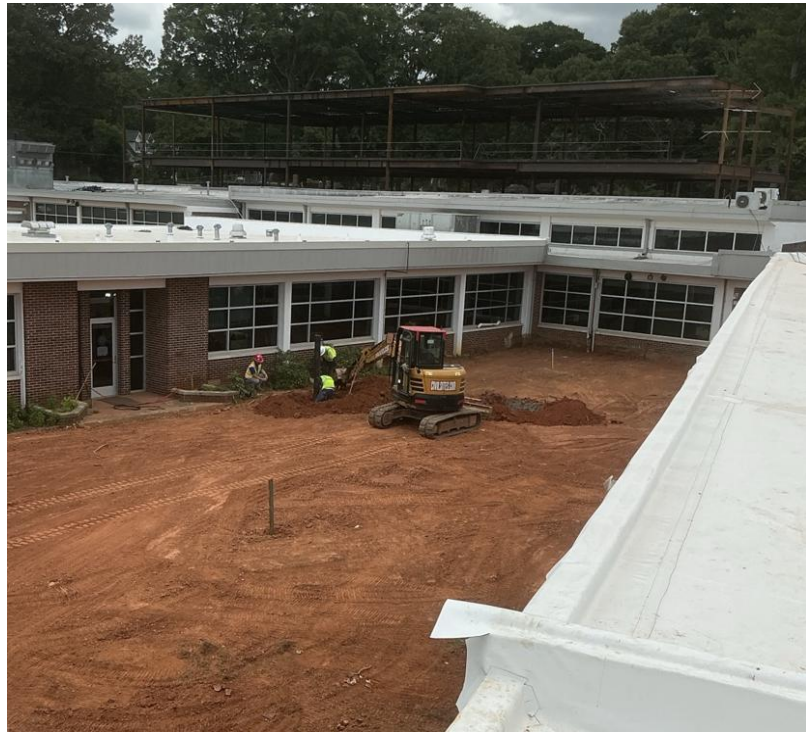
Installation of utilities at courtyards
