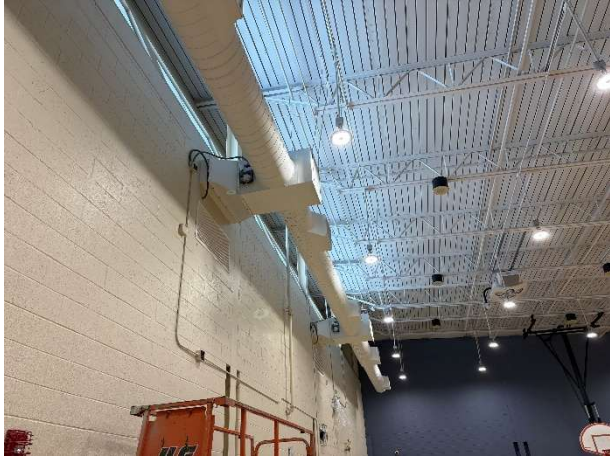
Spiral Duct Painted and HVAC System Start-up Complete
