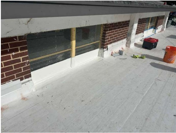
Roof Replacement Complete on West Side of Roof
