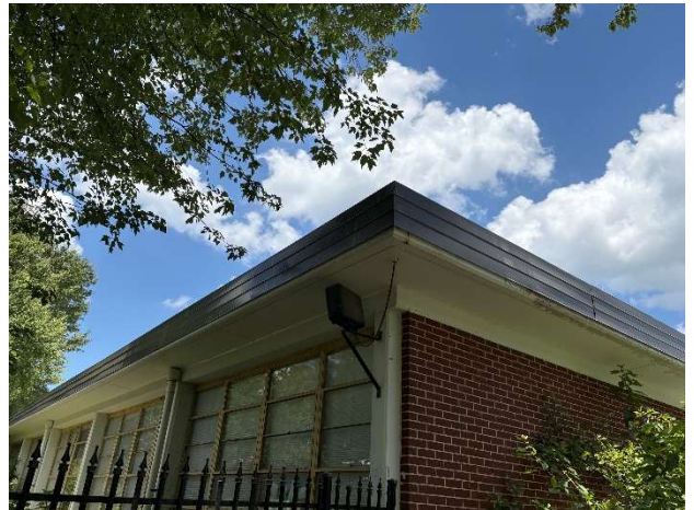
Roof Edge Metal Installation Complete
