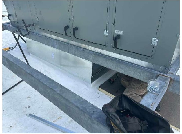
Mechanical Shroud Replacement Complete
