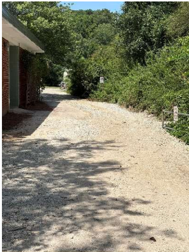
Exterior Punch Work Complete
