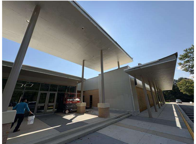
Waterproofing at bus canopy
