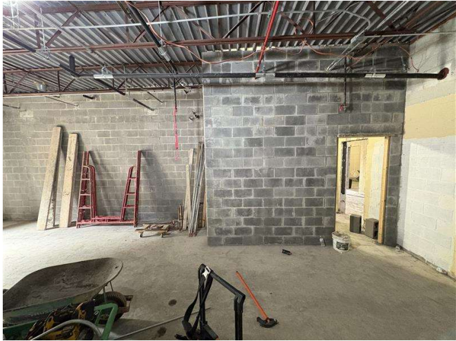
New classroom and restroom walls built
