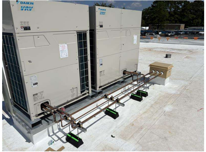
Rooftop units set and being connected
