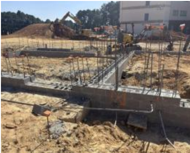
Foundation Wall CMU at Zone F
