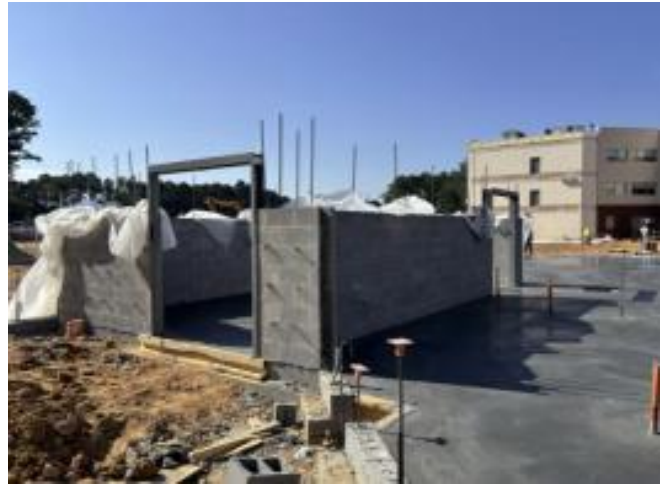
CMU at Stair 2
