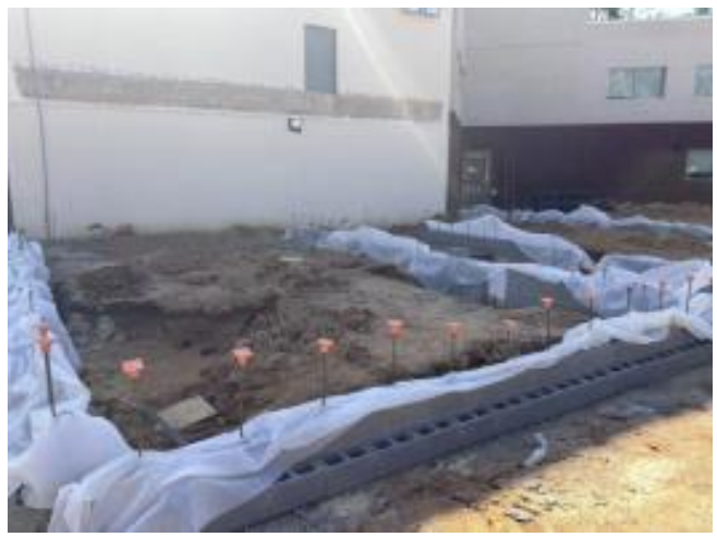
Foundation Wall CMU at Zone G
