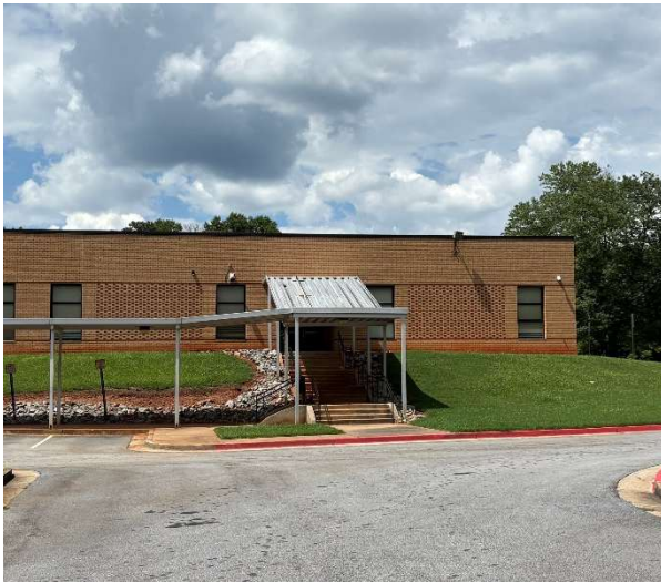
Roof Edge Metal Complete (South Side)
