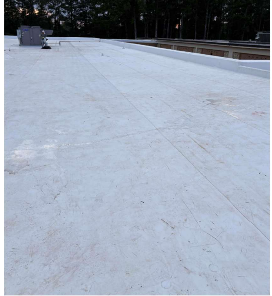
TPO Membrane Installation Complete (North Side)
