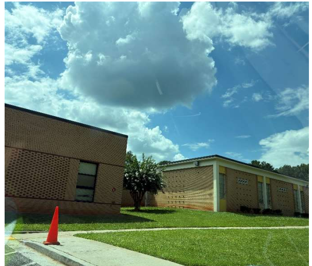
Roof Edge Metal Complete (East Side)
