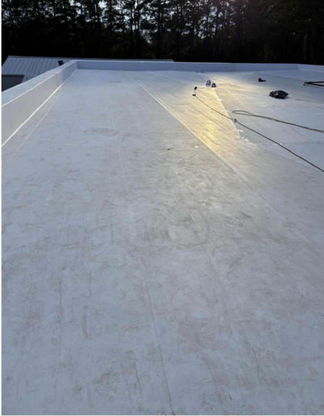
TPO Membrane Installation Complete (South Side)
