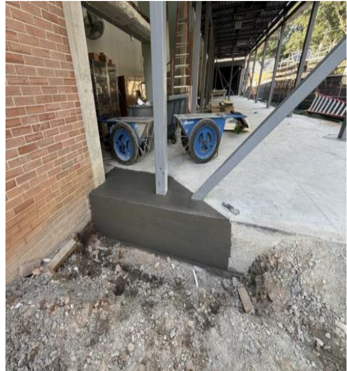
Concrete in-fill at cafeteria expansion
