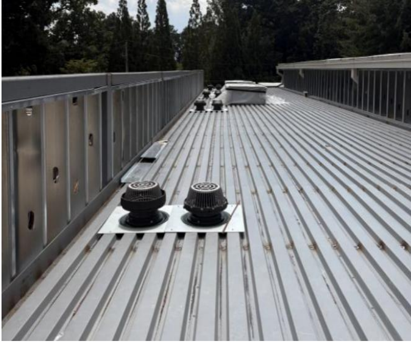
Roof drains and decking at cafeteria expansion
