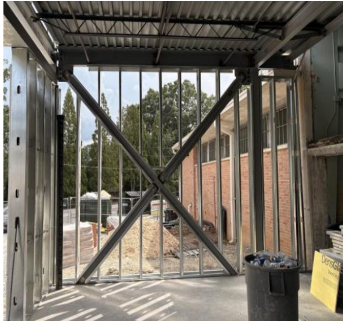
Metal Framing at cafeteria expansion
