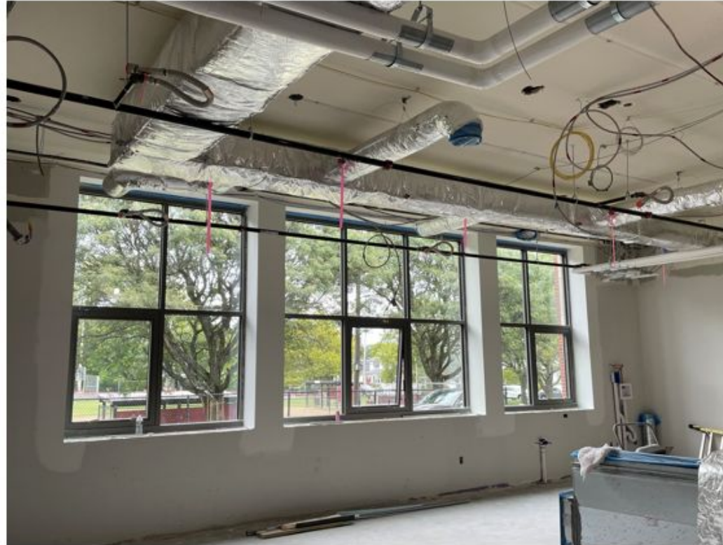
1st floor corridor - renovated area
