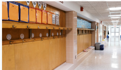
CORRIDOR CEILING REPLACEMENT
