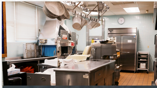
KITCHEN RENOVATION (NEW COOLER & FREEZER)
