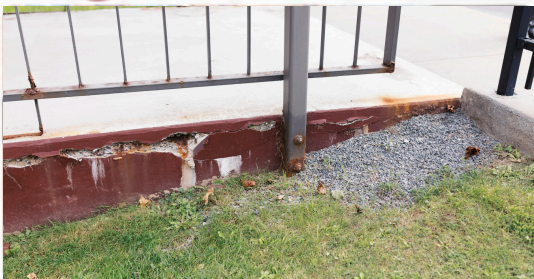
ENTRANCE BRIDGE RESTORATION
