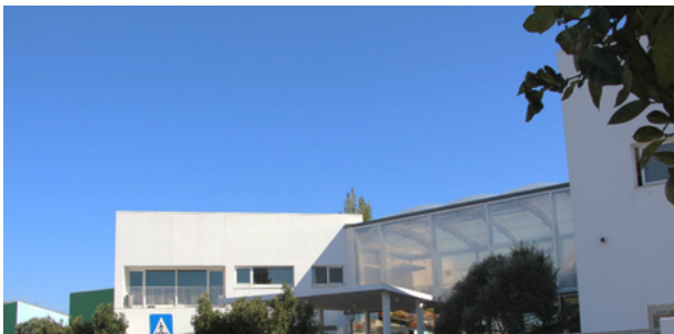
Main entrance (Atrium) [Years 3 to 6]
