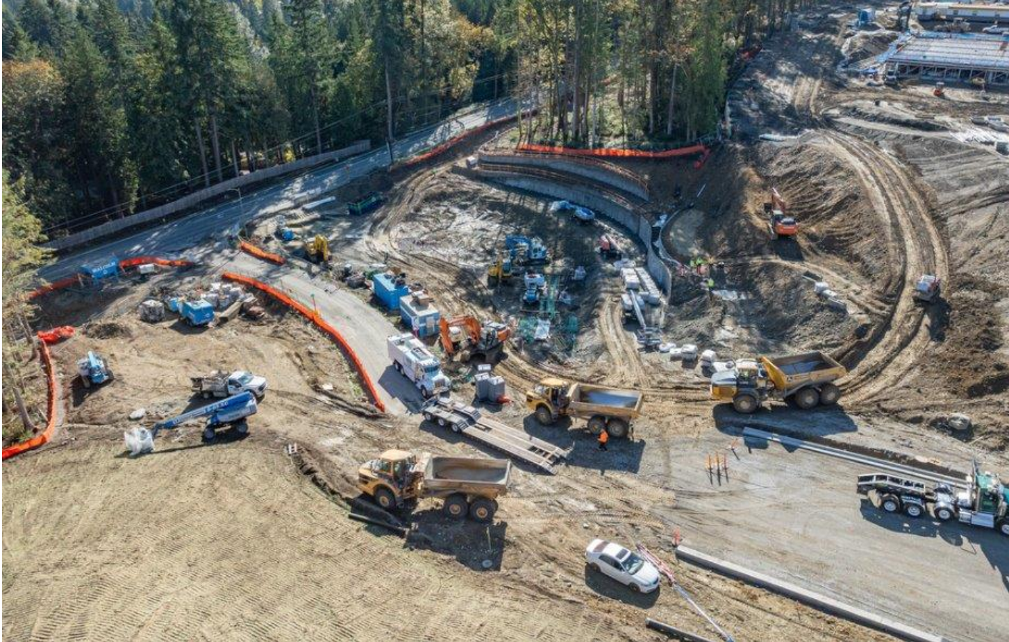
View of the main entrance being graded and retaining walls installed (drone photo taken 10/12/26)
