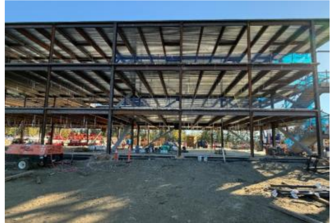
View of the main building classroom bar fully erected with decking and stairs in place (photo taken 10/7/26)
