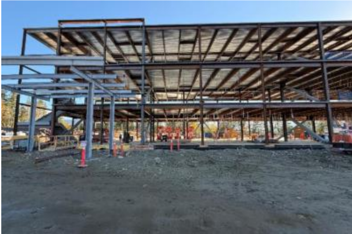
View of the main building classroom bar fully erected with decking and stairs in place (photo taken 10/7/26)
