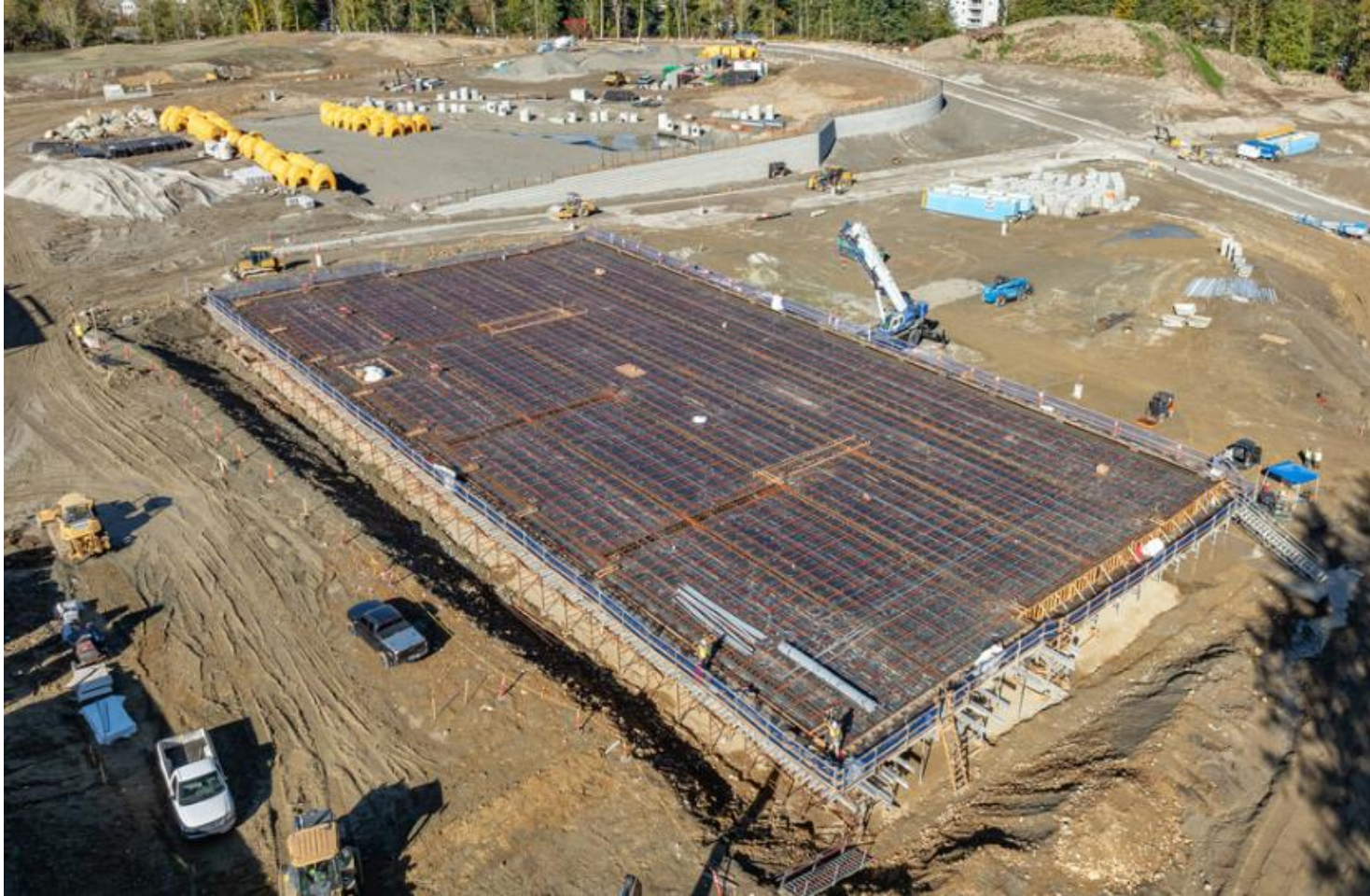
View of the parking garage slab and post-tension slab preparation nearly complete (drone photo taken 10/12/26)
