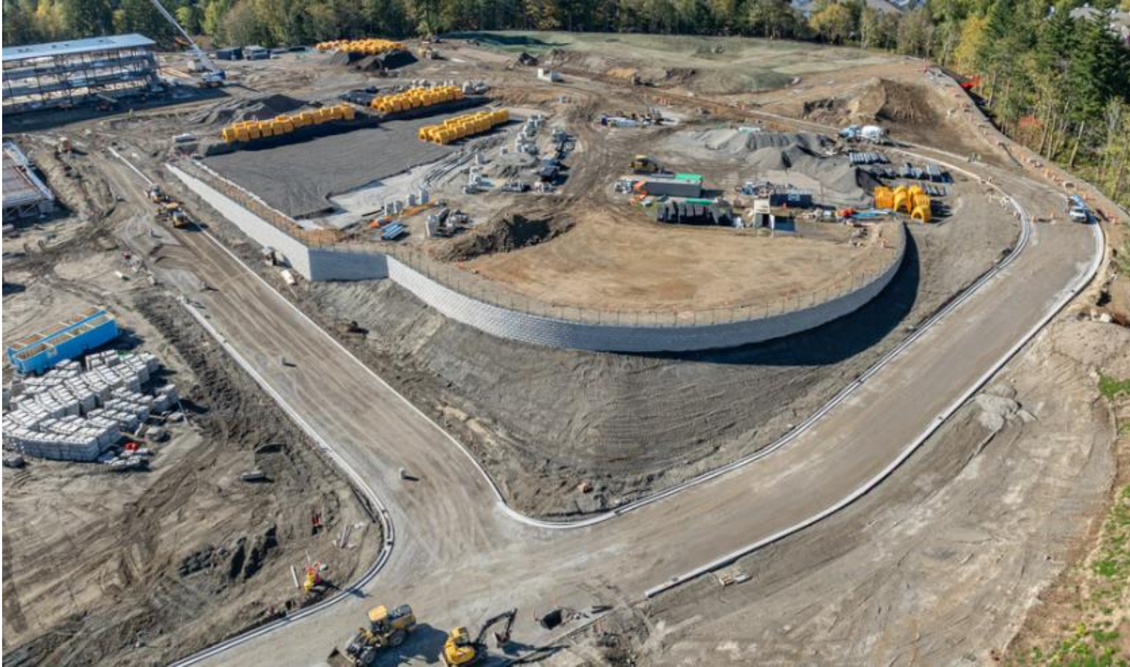
Aerial view of the future sports field area with retaining wall completed and underground storm water system being prepared for structure installation (drone photo taken 10/12/26)
