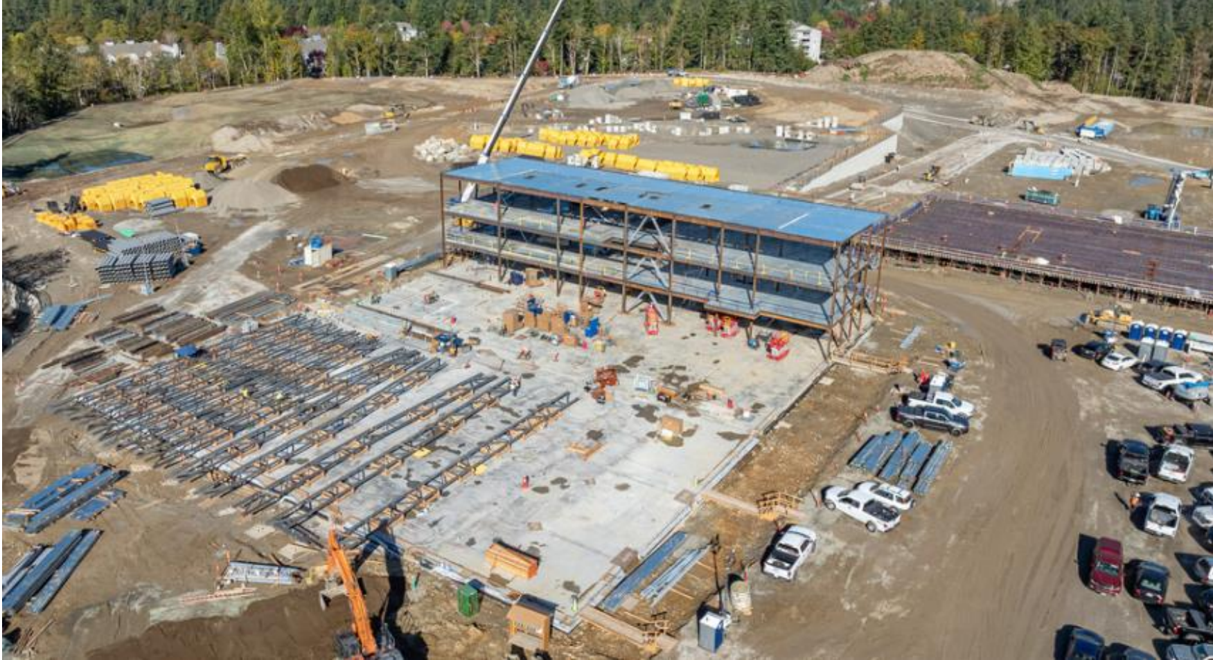
View of the main building with steel erection well underway (drone photo taken 10/12/26)
