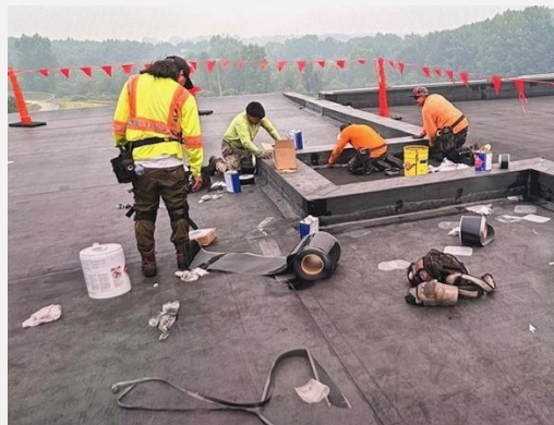
High School Roofing Project.
