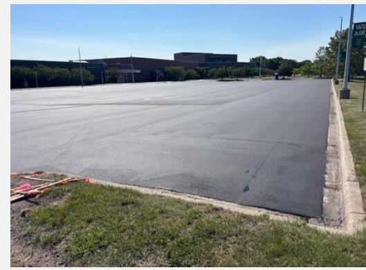
High School Paving Project.
