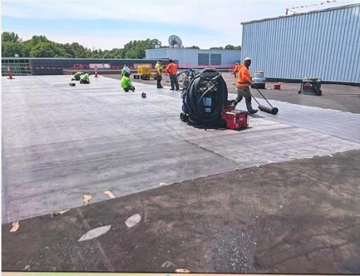
High School Roofing Project.
