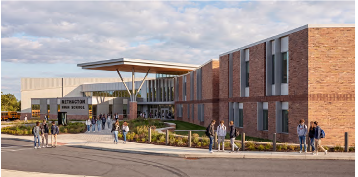
View of Classroom Wing / Main Entrance
