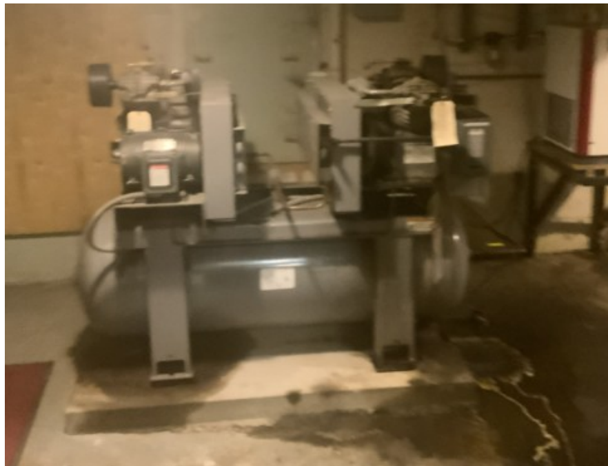
Existing Pneumatic Control Air Compressors
