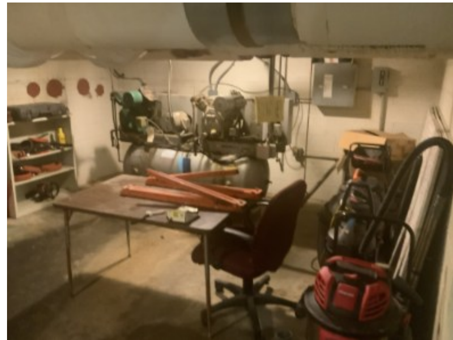
Existing Pneumatic Control Air Compressors
