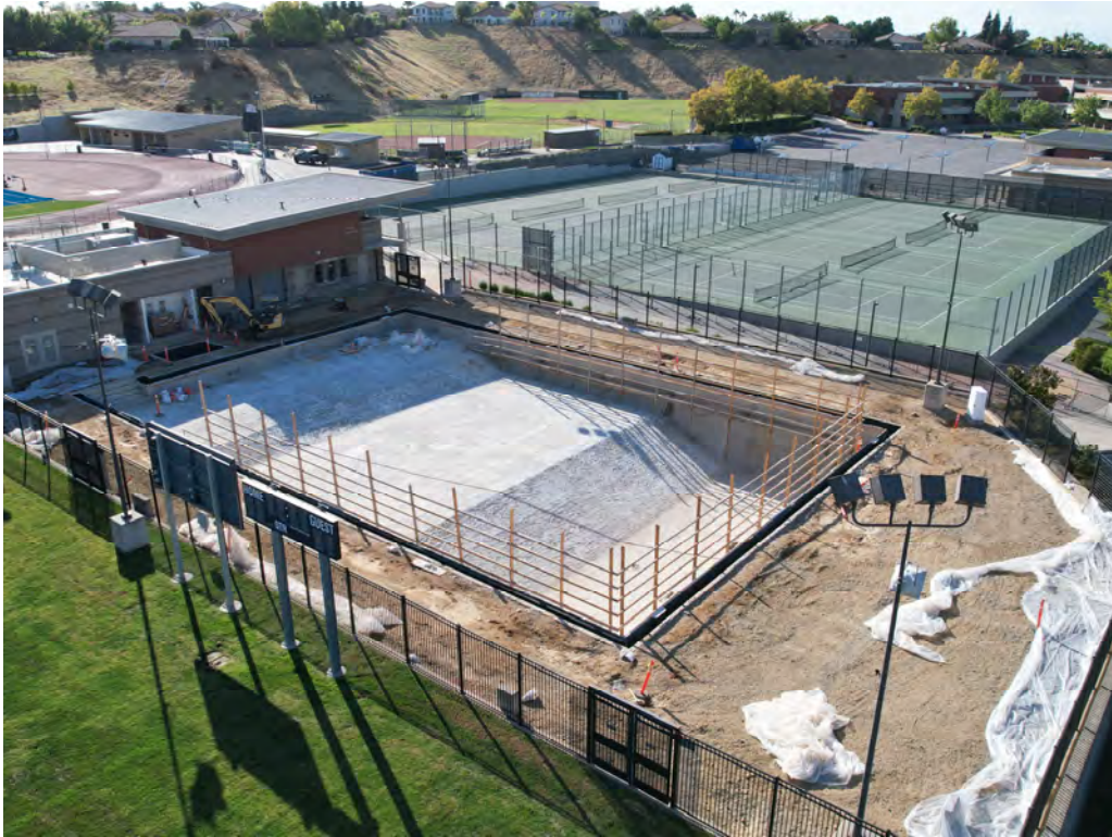
Photo 8 — View to the southwest of the pool area (under construction) in the central portion of the site. Fill (part of the cap system) is shown around the pool area.
