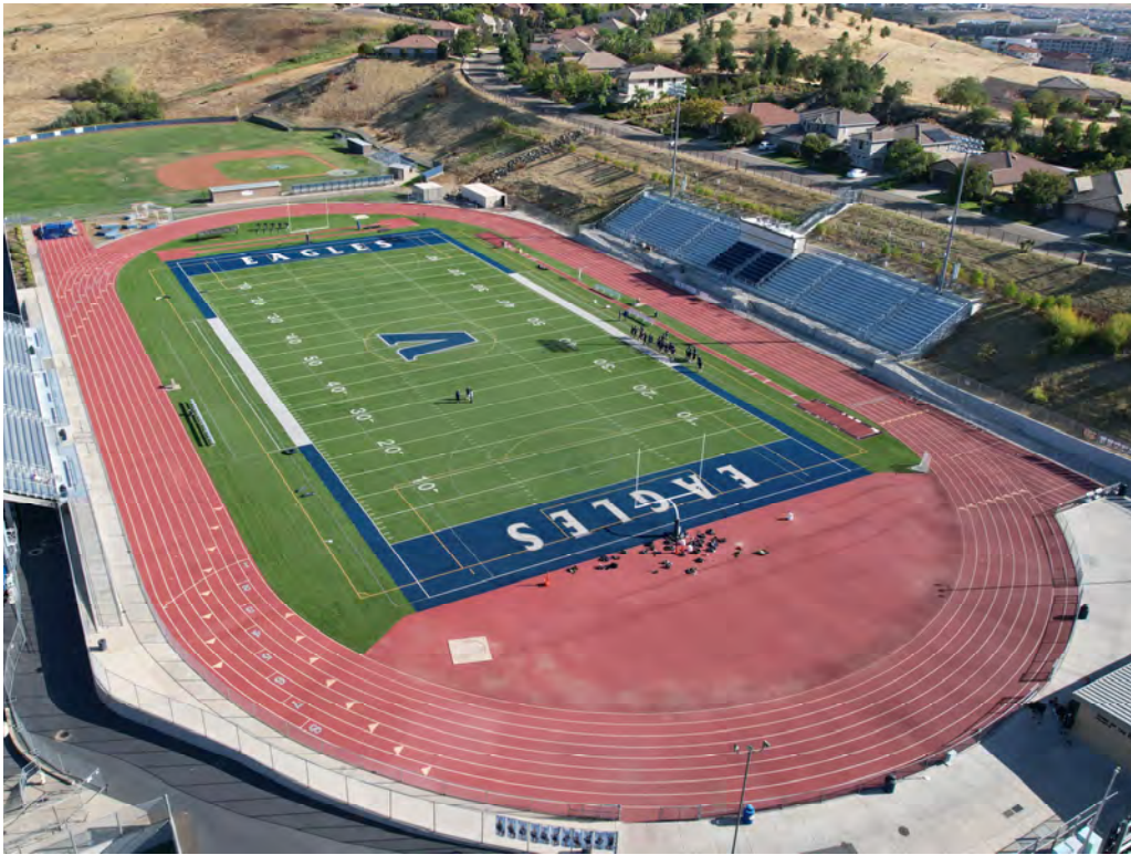
Photo 9 — View to the southeast of the football field and track in the southern portion of the site.
