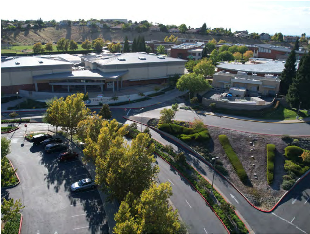
Photo 1 — View to the west of traffic and fire lanes and Buildings B and C in the northeastern portion of the site.
