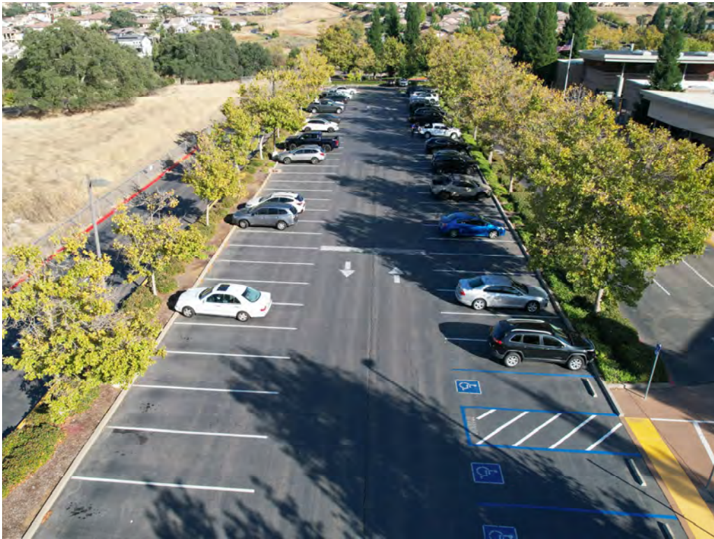
Photo 4 — View to the east of Parking Lot 2 in the northern portion of the site.
