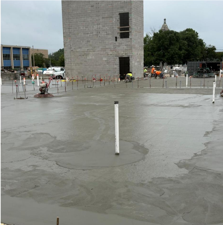
Classroom Area, Slab on Grade Concrete
