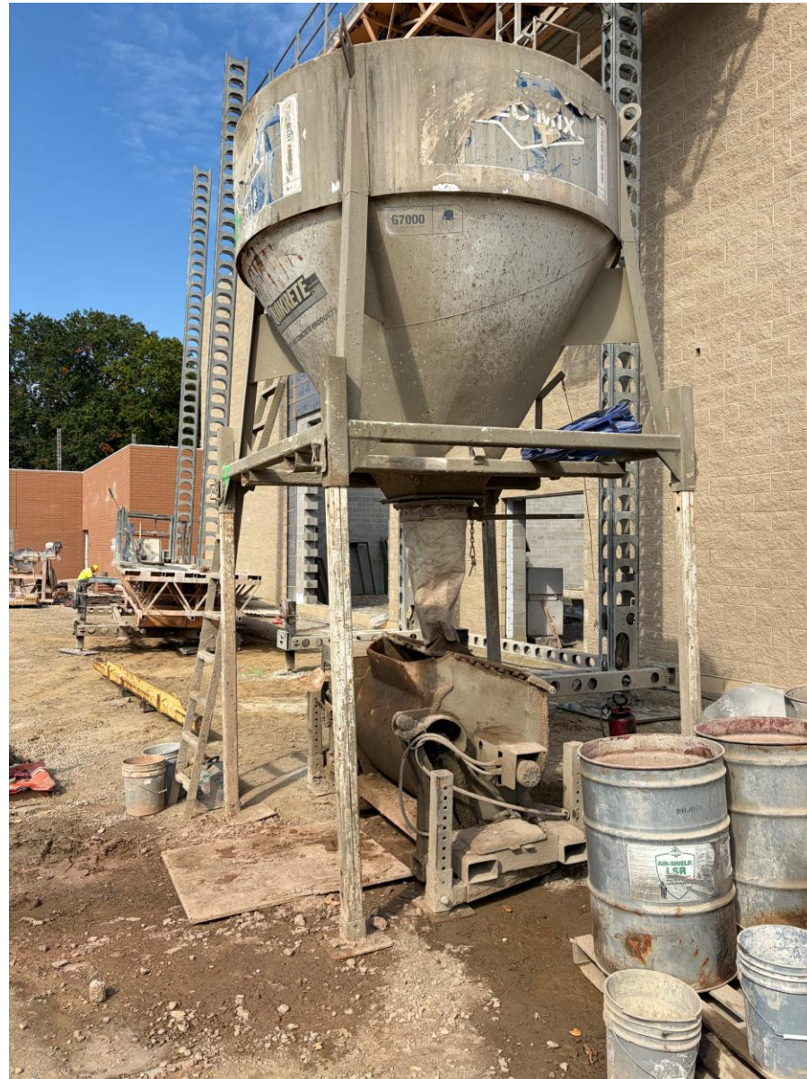
HOPPER AND DUST BAFFLES
