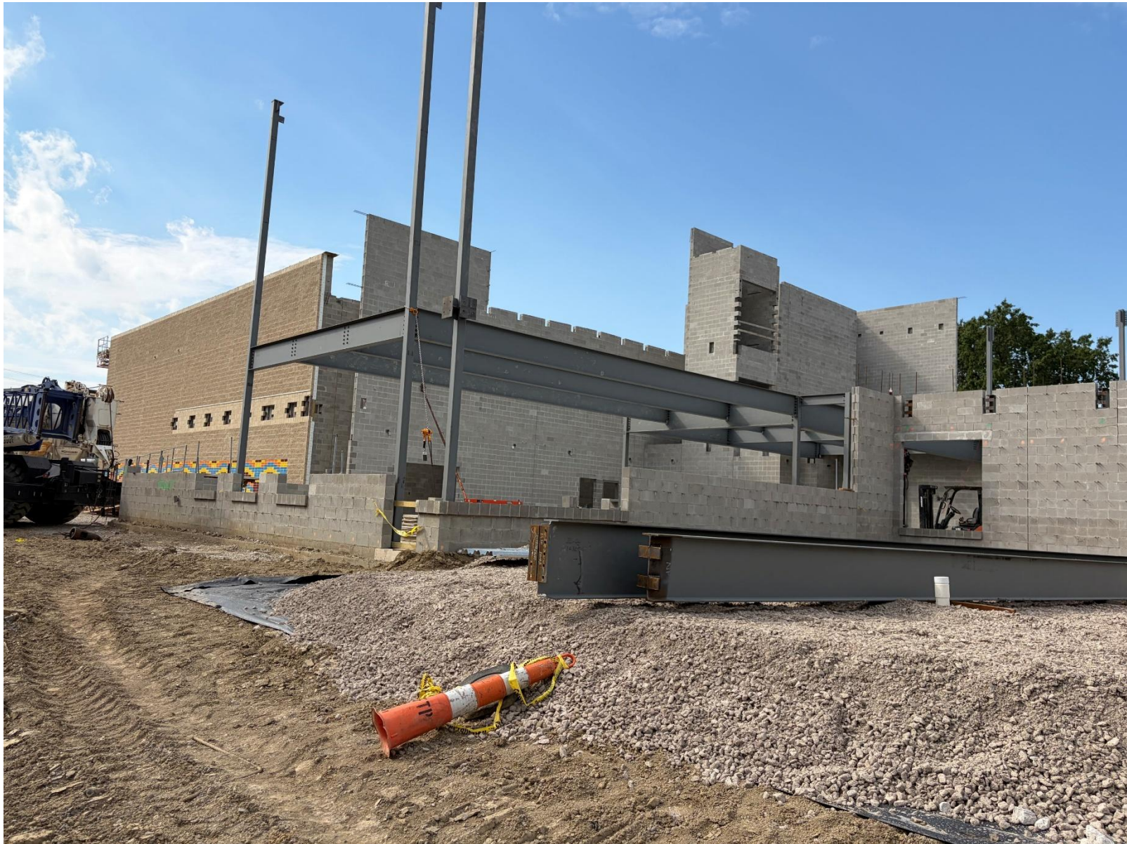
EAST ELEVATION – GYM WALL AND ADMIN AREA STEEL
