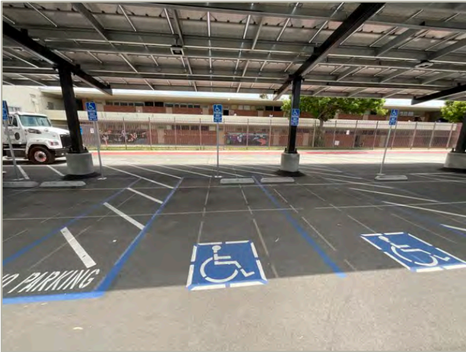
OVERVIEW OF ACCESSIBLE PARKING AREA
