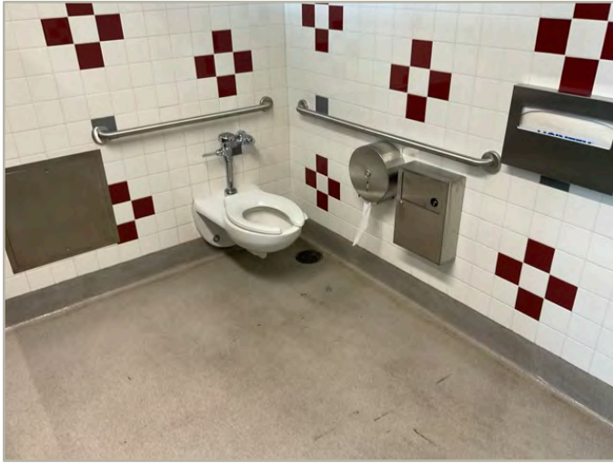
TOILET STALL OVERVIEW
