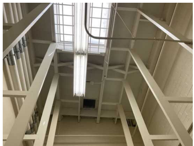
6 - WALL AND ROOF STRUCTURE
