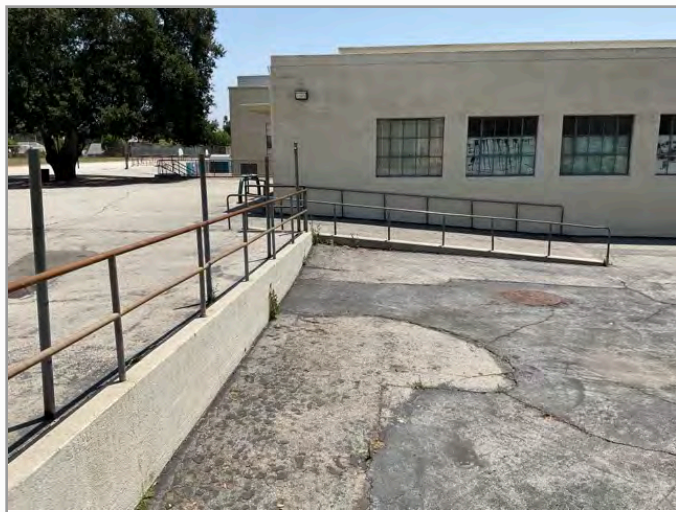
Accessible route to playground
