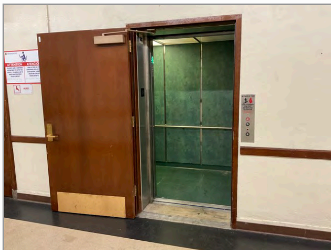
Lobby looking at cabs
