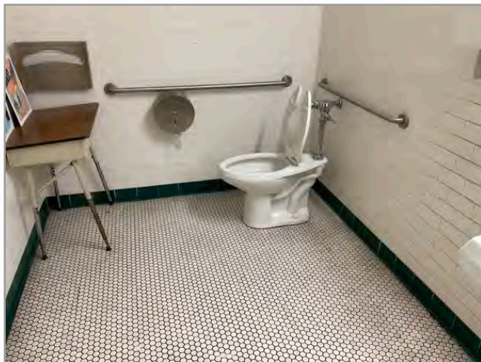
Toilet stall overview
