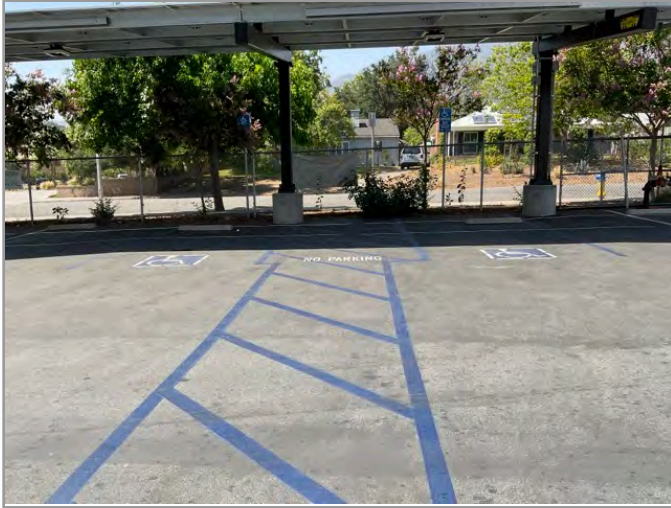
Overview of accessible parking area
