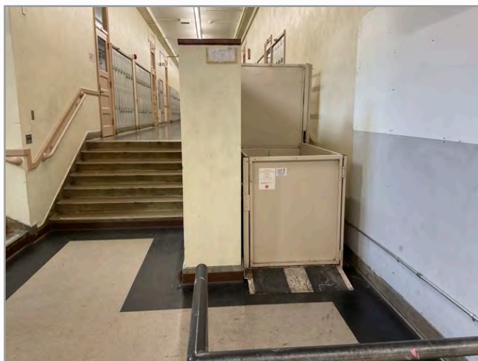
Accessible interior path (lift)
