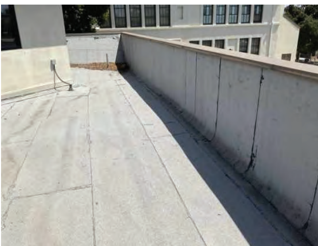
5 - ROOFING OF LIBRARY
