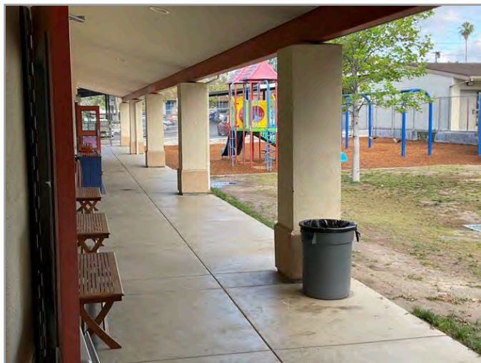
Accessible route to playground/pool
