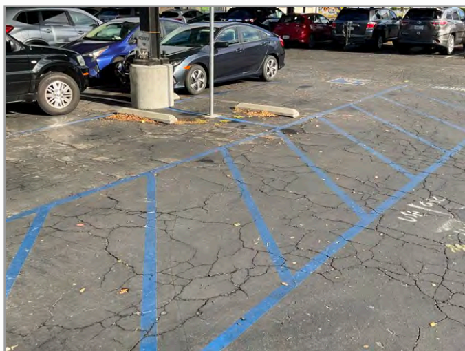
Overview of accessible parking area
