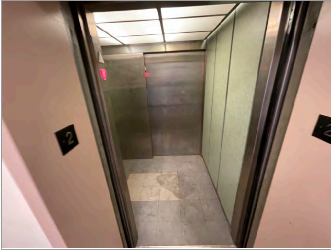
Lobby looking at cabs (with doors open)
