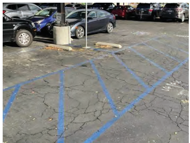
6 - OVERVIEW OF ACCESSIBLE PARKING AREA
