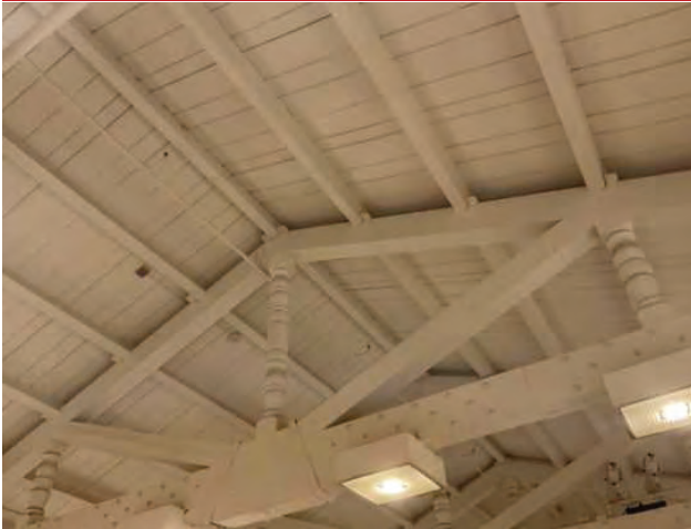
19 - WOODEN TRUSS ROOF STRUCTURE
