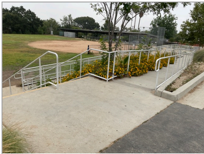
Accessible route to playground
