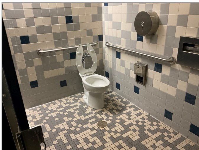
Toilet stall overview
