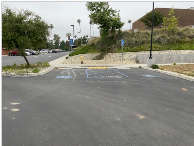
Overview of accessible parking area
