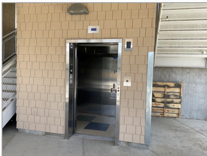
Lobby looking at cabs
