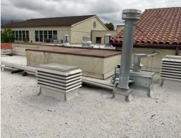
7 - PRIMARY ROOF OVERVIEW
