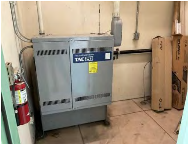
21 - ELEVATOR HYDRAULIC PUMP
