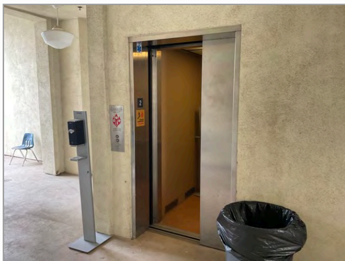
Lobby looking at cabs
