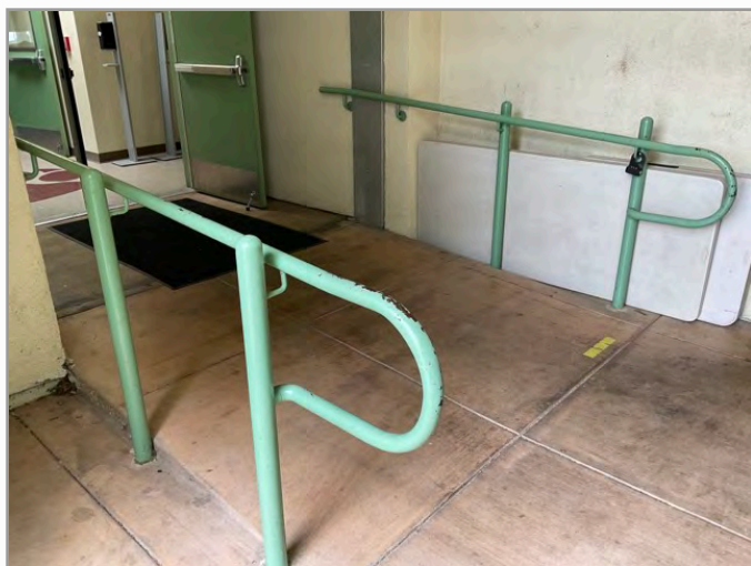
Accessible interior path ramp
