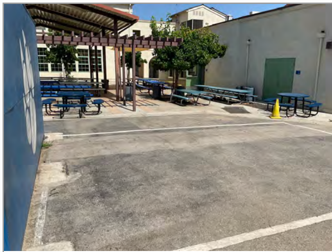
Accessible route to playground
