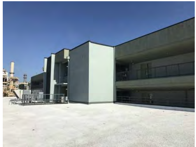
10 - HIGH SCHOOL ROOFING
