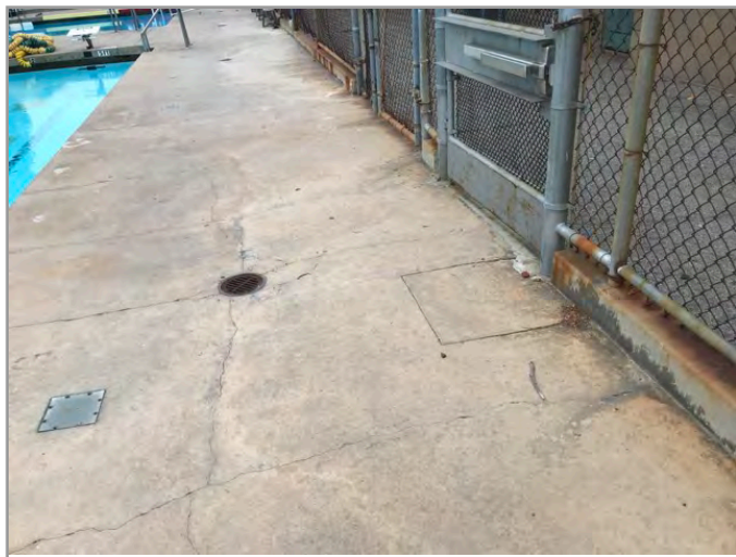
ACCESSIBLE ROUTE TO POOL
