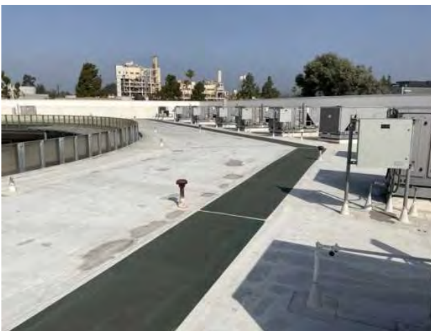
11 - MIDDLE SCHOOL ROOFING
