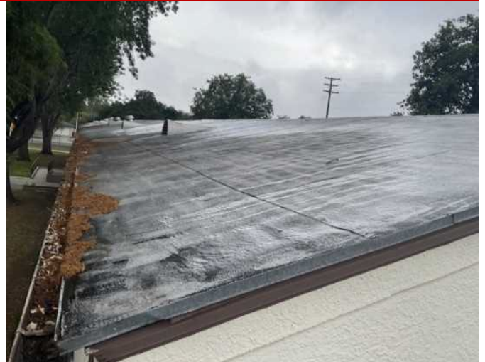
8 - MODIFIED BITUMINOUS ROOF
