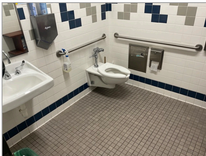
Toilet stall overview
