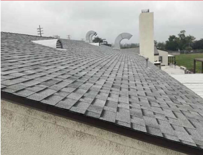
7 - ASPHALT SHINGLES ROOF
