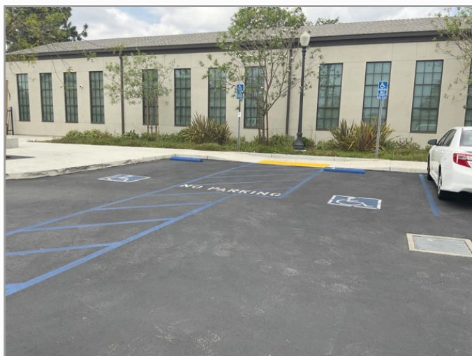
Overview of accessible parking area
