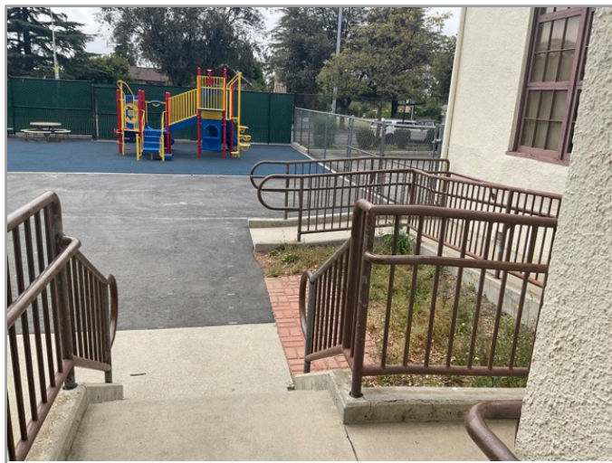
Accessible route to playground
