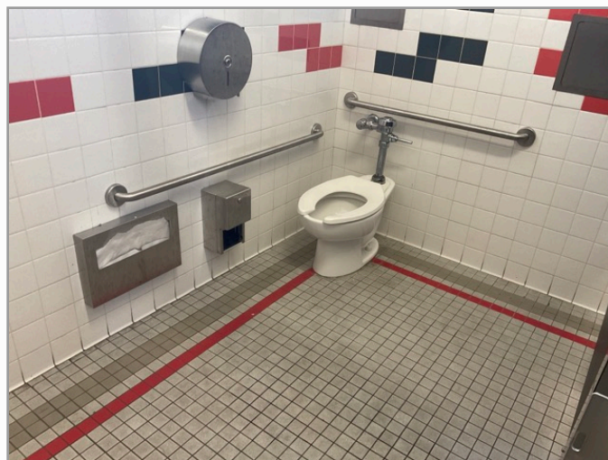
Toilet stall overview
