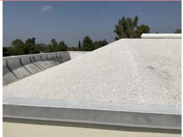
8 - SECONDARY ROOF OVERVIEW
