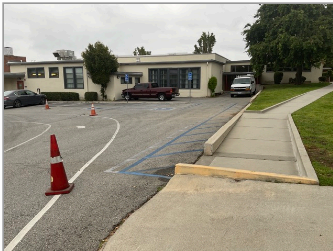
Overview of accessible parking area
