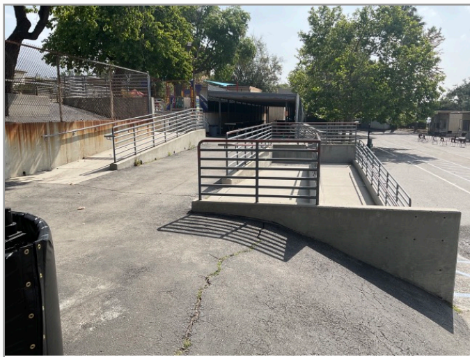
Accessible route to playground
