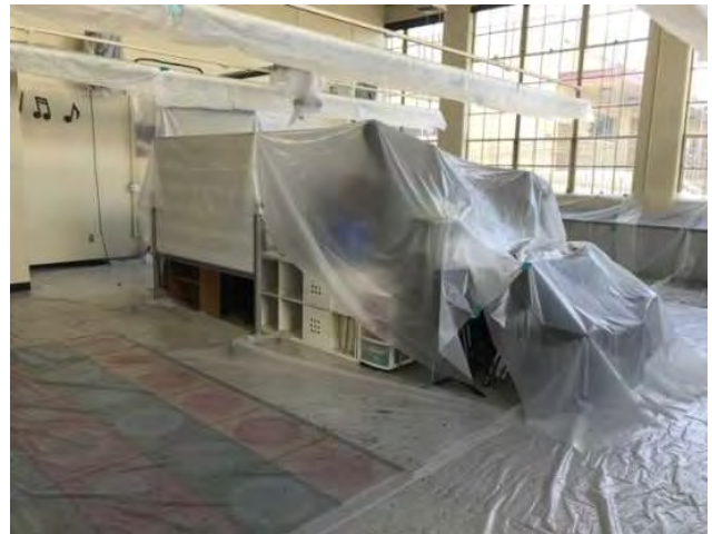
40 - BUILDING C UNDER CONSTRUCTION
