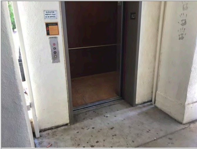
LOBBY LOOKING AT CABS (WITH DOORS OPEN)
