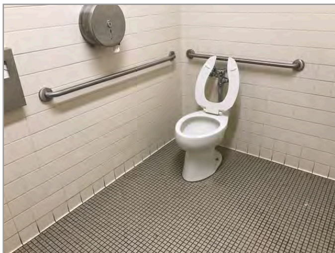
TOILET STALL OVERVIEW
