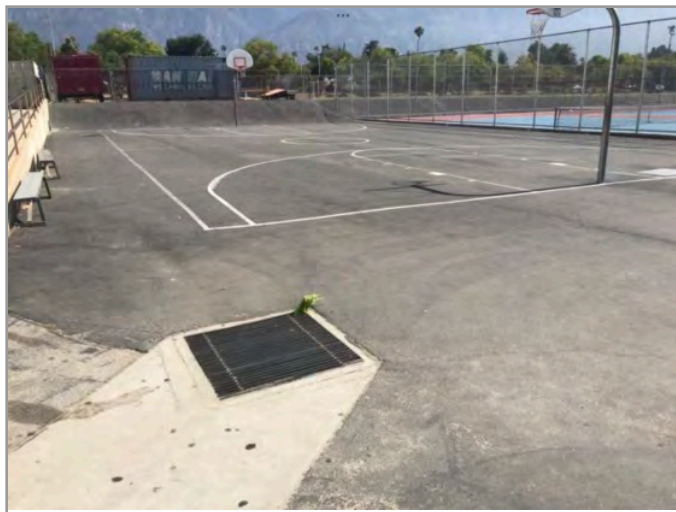
ACCESSIBLE ROUTE TO PLAYGROUND
