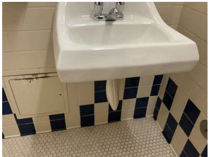
24 - SINK STAFF BUILDING A
