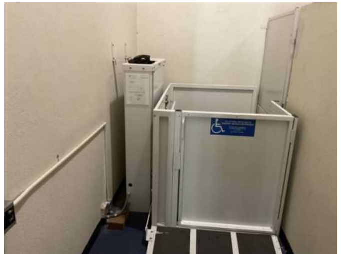
28 - VERTICAL LIFT BUILDING A
