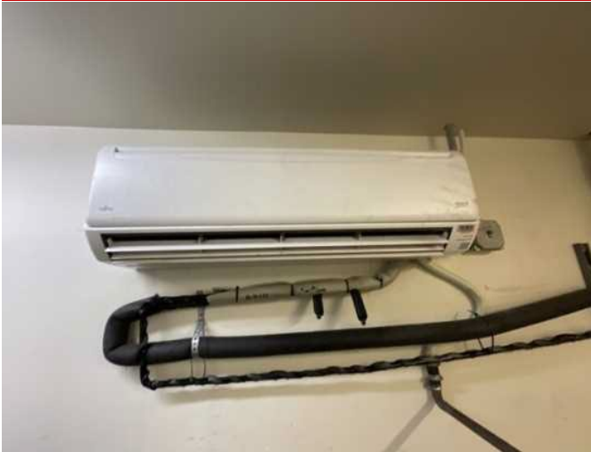
31 - SPLIT SYSTEM DUCTLESS EVAPORATOR
