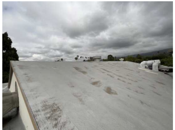
10 - BUILDING A ROOFING
