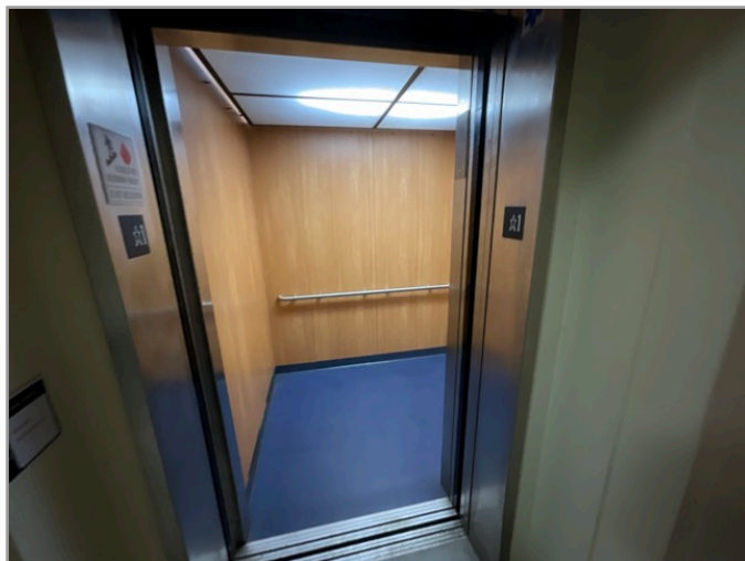
Lobby looking at cabs (with doors open)
