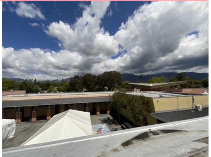
20 - OVERVIEW OF COURTYARD
