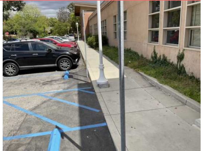
8 - CLOSE-UP OF ACCESSIBLE PARKING
