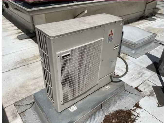
32 - SPLIT SYSTEM DUCTLESS CONDENSER
