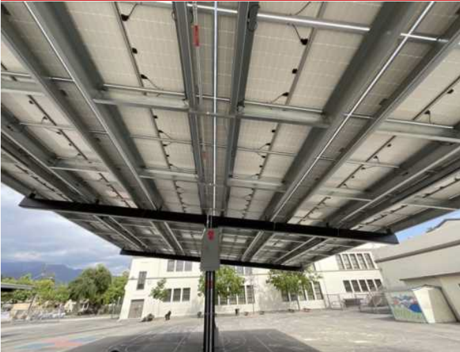
7 - SOLAR PANEL SHADE APPARATUS
