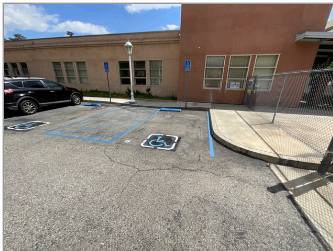
Overview of accessible parking area
