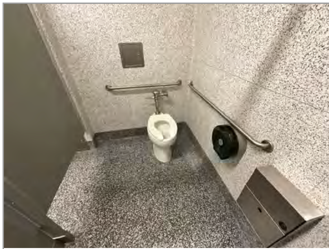
TOILET STALL OVERVIEW
