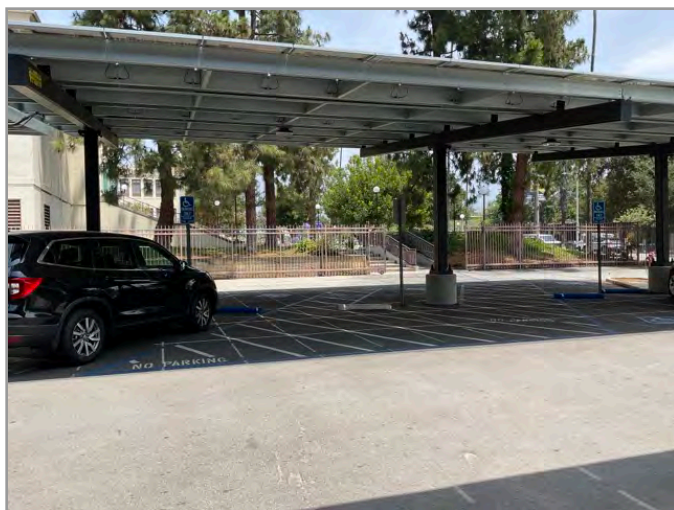
OVERVIEW OF ACCESSIBLE PARKING AREA
