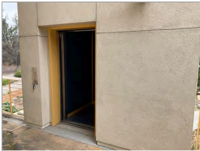
LOBBY LOOKING AT CABS (WITH DOORS OPEN)
