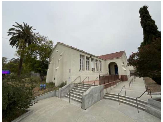
10 - FACADE OVERVIEW - OLD
