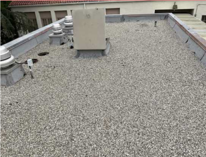
13 - SECONDARY ROOFING OVERVIEW
