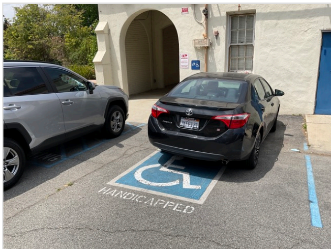
OVERVIEW OF ACCESSIBLE PARKING AREA
