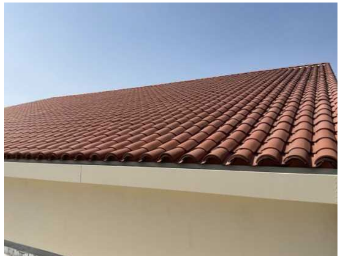
12 - PRIMARY ROOFING OVERVIEW
