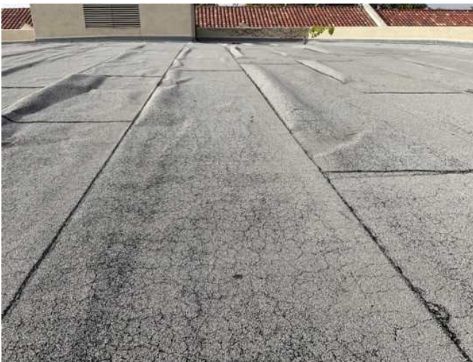
9 - MODIFIED BITUMINOUS ROOF
