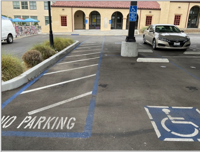
Overview of accessible parking area
