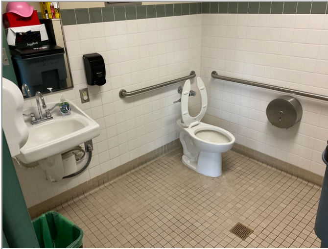
Toilet stall overview
