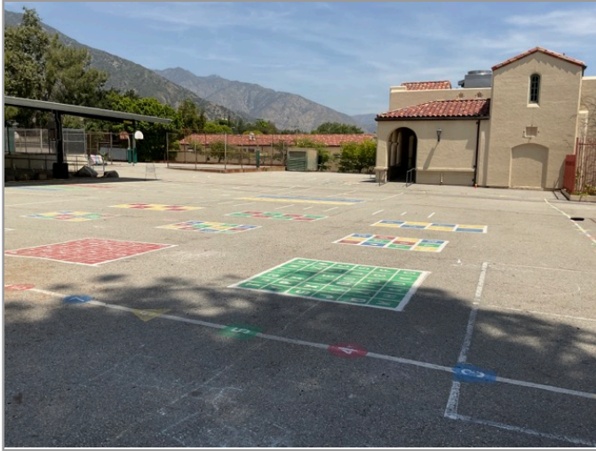
Accessible route to playground
