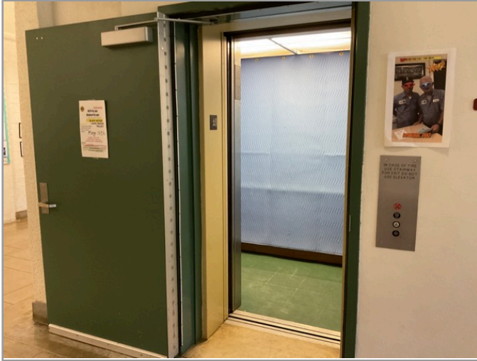
Lobby looking at cabs (with doors open)
