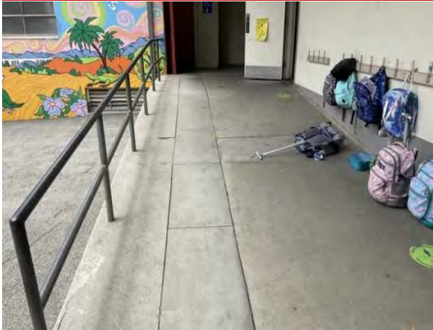
31 - RAMP TO MULTI-PURPOSE ROOM
