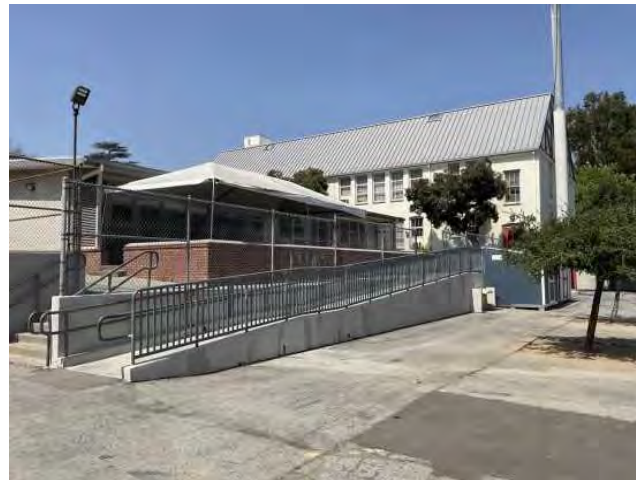
34 - RAMP TO PLAYGROUND
