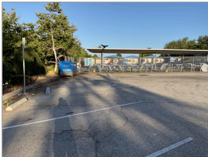
Overview of accessible parking area
