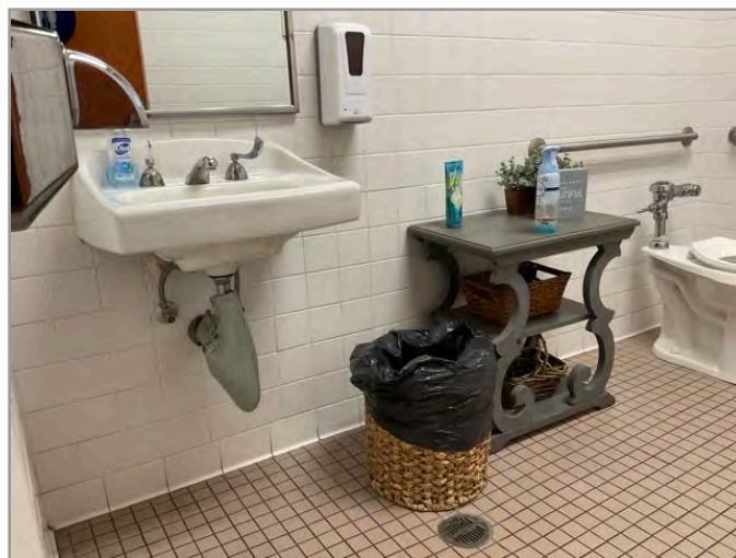
Sink and faucet handles
