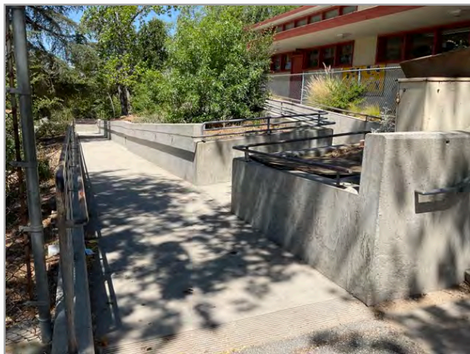
Accessible route to playground
