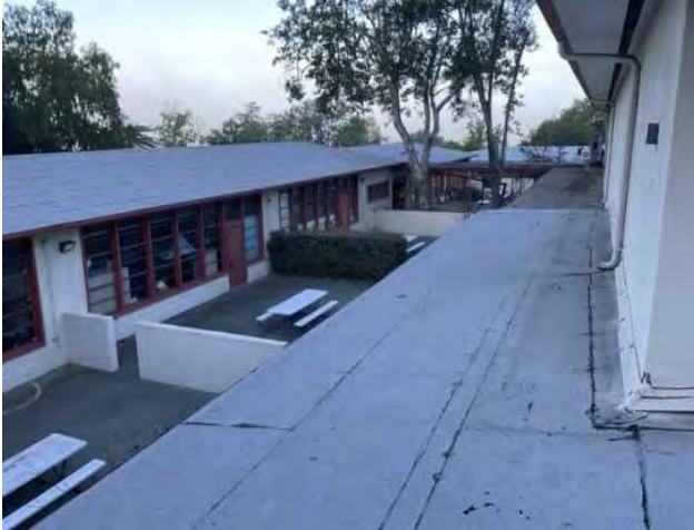
7 - PRIMARY ROOF OVERVIEW
