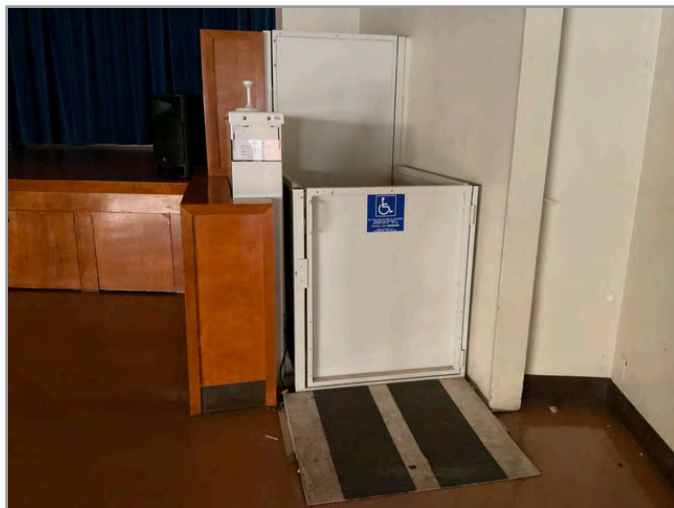
Accessible interior path (lift)
