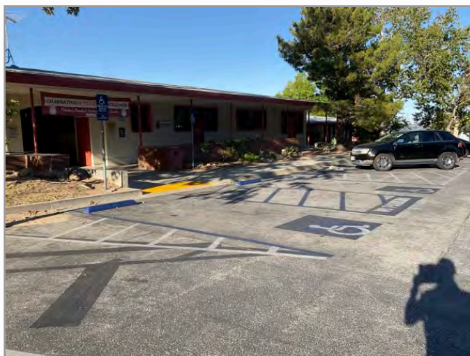
Overview of accessible parking area
