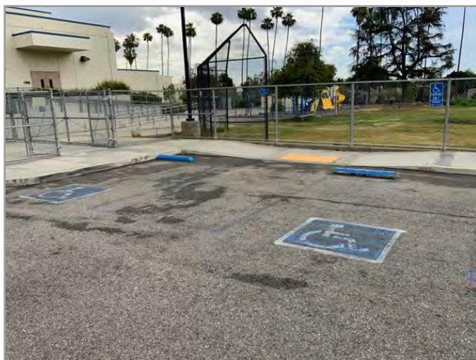
OVERVIEW OF ACCESSIBLE PARKING AREA
