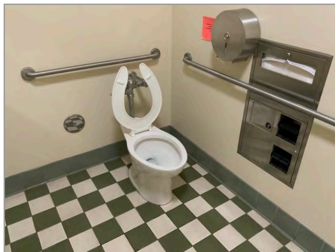
TOILET STALL OVERVIEW
