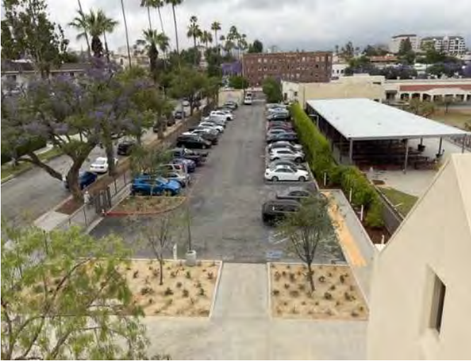
37 - PRIMARY PARKING AREA
