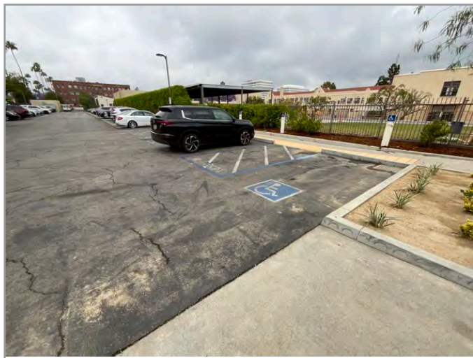
OVERVIEW OF ACCESSIBLE PARKING AREA
