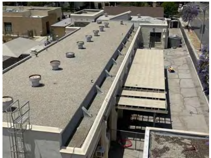
12 - PRIMARY ROOF OVERVIEW
