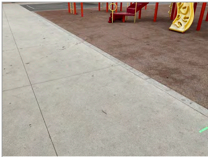
ACCESSIBLE ROUTE TO PLAYGROUND
