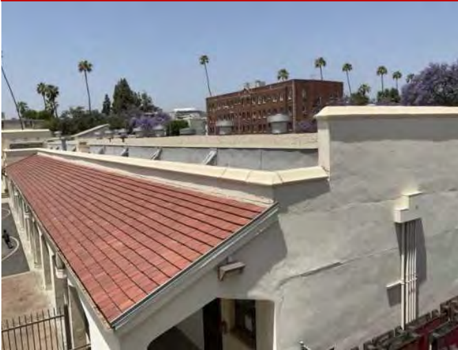
13 - SECONDARY ROOF OVERVIEW
