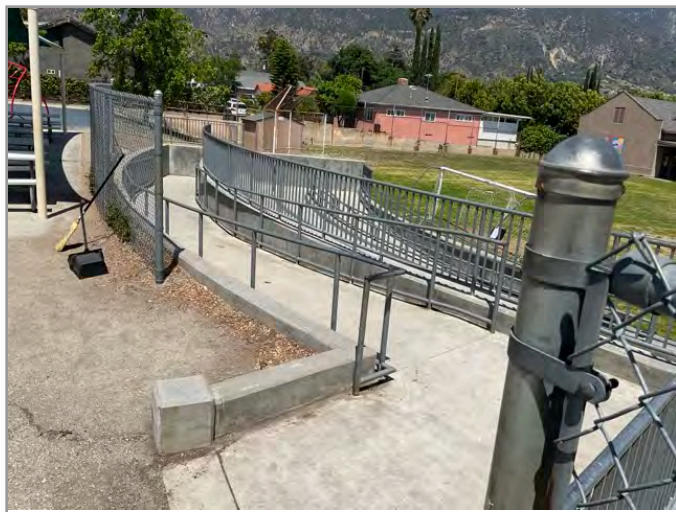
Accessible route to playground
