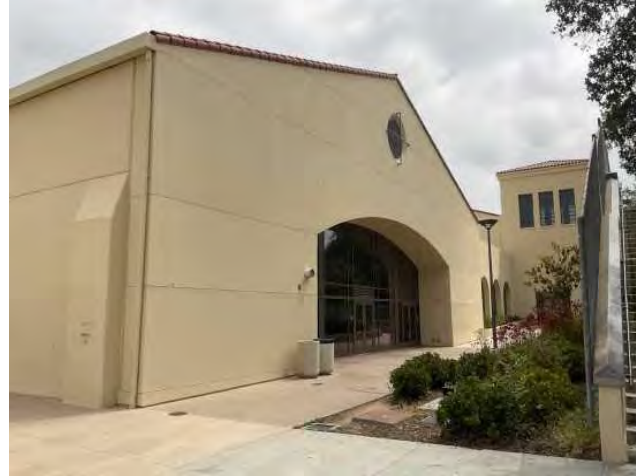
14 - PAINTED EXTERIOR STUCCO
