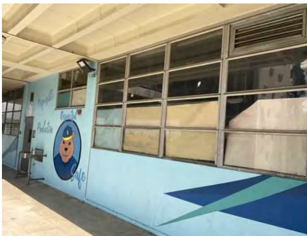
17 - METAL FRAMED WINDOWS
