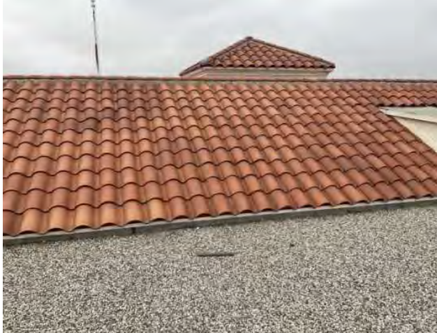
13 - CLAY TILE ROOFING
