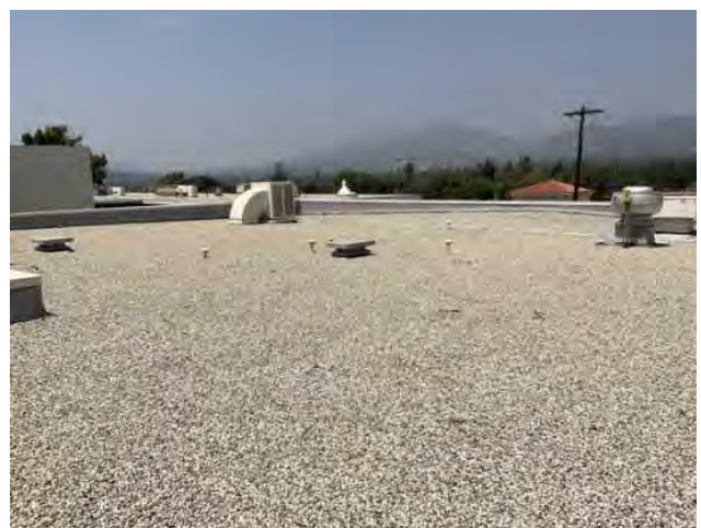
12 - MODIFIED BITUMINOUS ROOFING
