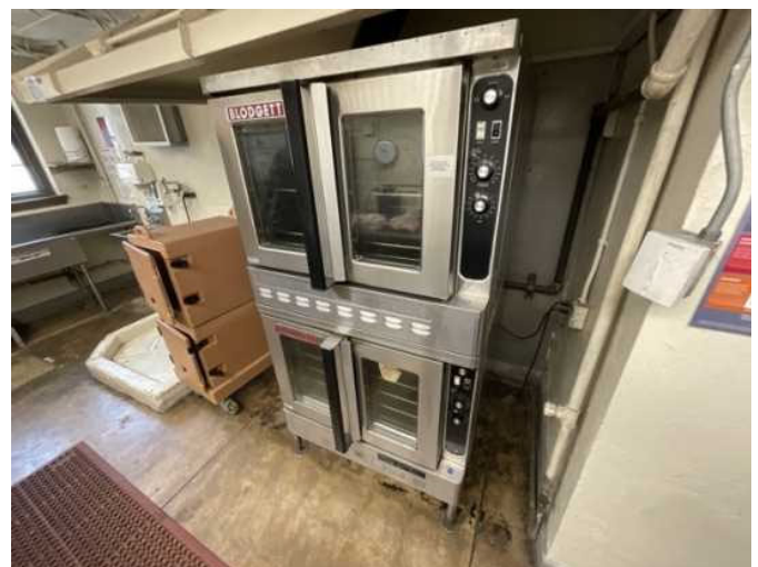
30 - COMMERCIAL KITCHEN EQUIPMENT
