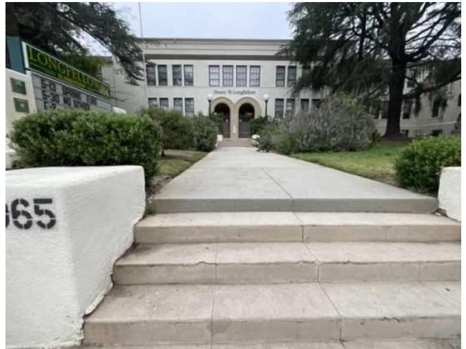
34 - STAIRS AND CONCRETE WALKWAYS
