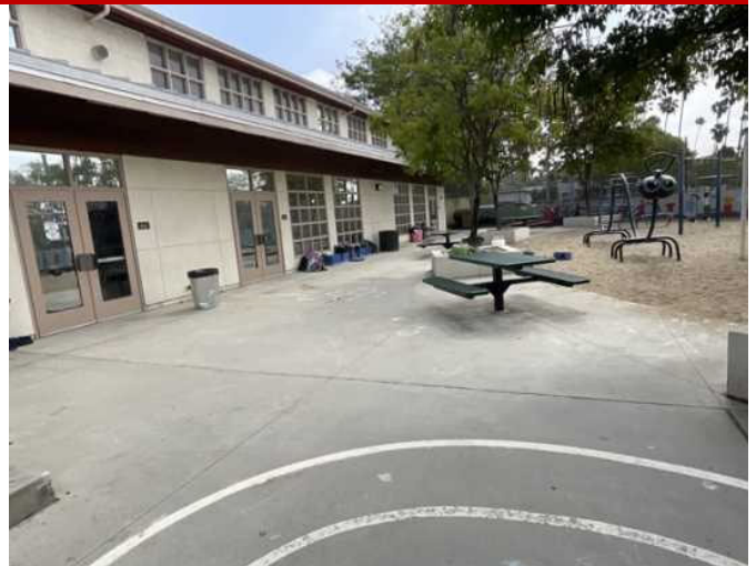
8 - EXTERIOR WINDOWS AND DOORS
